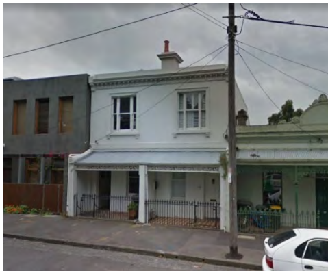
Figure 15 36 Macarthur Place North (HO1) Source: Streetview
