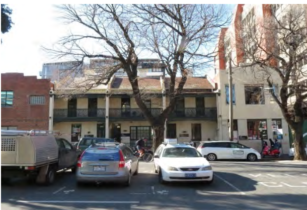
Figure 11 Terrace row, 18-22 Cardigan Street (HO35) Source: Lovell Chen
