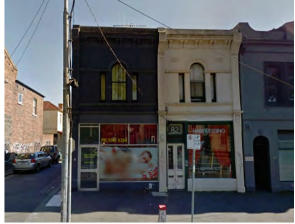
Figure 12 82-84 Elgin Street, Carlton (HO1) Source: Google Streetview
