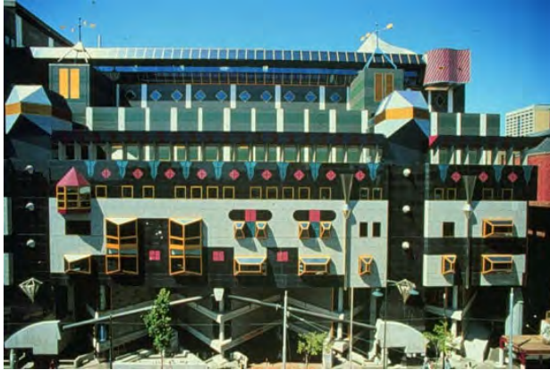
Figure 14 RMIT Building 8, 360 Swanston Street, Melbourne Source: http://architecture.rmit.edu.au/projects/r
