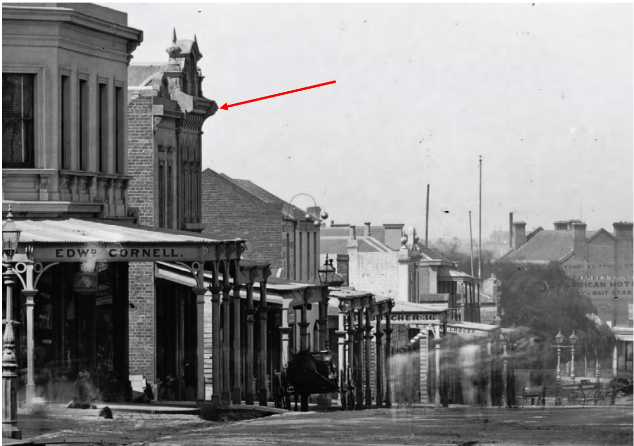
Figure 2 View south down Madeline Street from Queensberry Street, c. 1875, with the recently constructed subject buildings indicated Source: American & Australasian Photographic Company, a2825197, Mitchell Library, State Library of New South Wales
