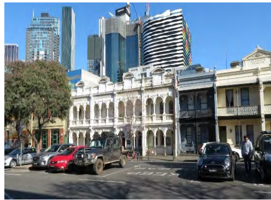
Figure 10 51-65 Cardigan Street, Carlton (HO27) Source: Lovell Chen
