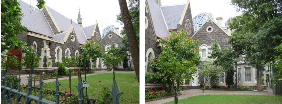
Figure 8 West side of church, showing adjoining presbytery Source: Lovell Chen
