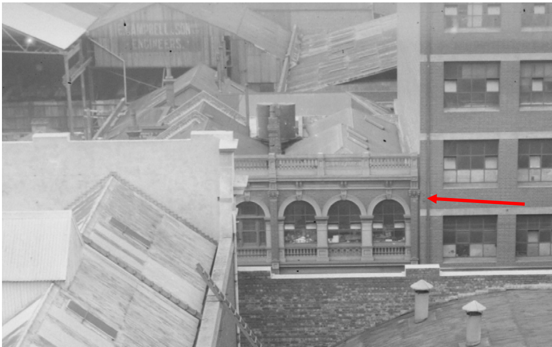
Figure 4 View across Carlton Brewery, c. 1920s, with top level of subject building visible Source: Walter Vears Collection, H99.149/65, State Library of Victoria
