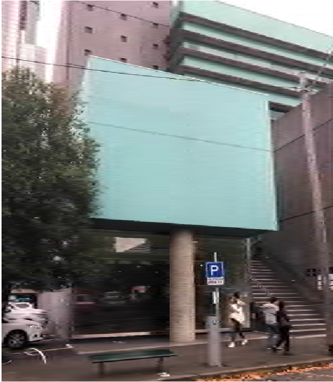
Figure 11 Detail of the mosaic tiled southern bay, resting on its single cylindrical column, with the staircase at right Source: Lovell Chen
