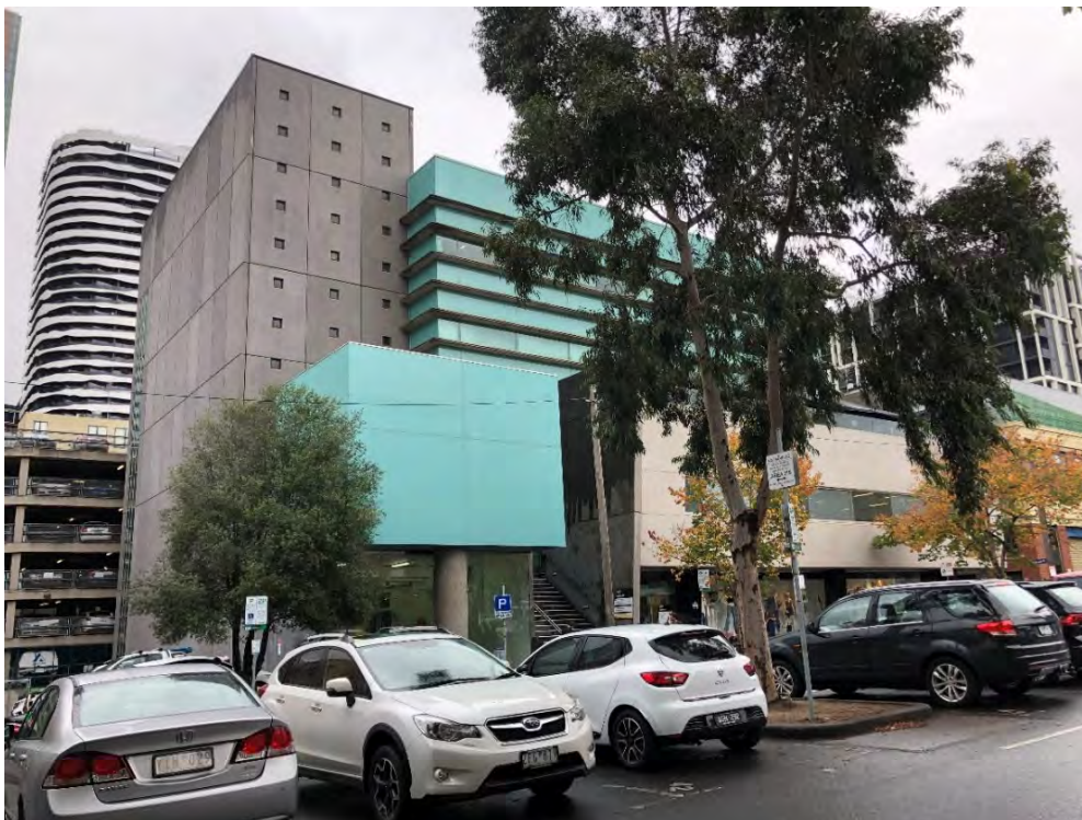
Figure 10 Subject building, viewed from the south; the grey concrete service block is at left, fronted by the southern bay clad in blue-green mosaic tiles Source: Lovell Chen
