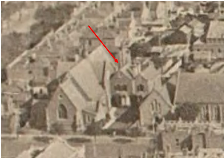
Figure 6 Oblique aerial view of church, 1927; note presbytery addition at right (indicated) Source: Airspy, H2501, State Library of Victoria
