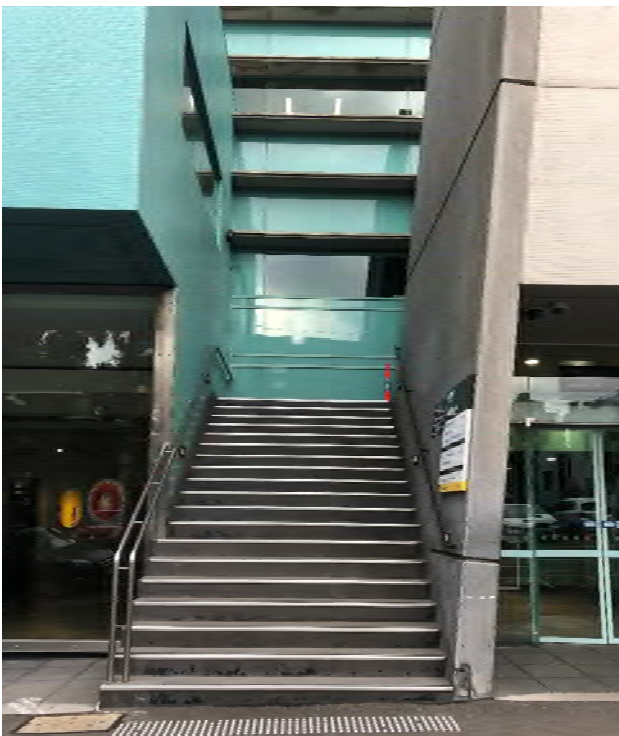
Figure 12 Detail of staircase, with angled south wall of the northern bay at right Source: Lovell Chen
