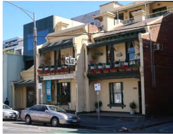
Figure 10 245-257 Cardigan Street, Carlton (HO34) Source: Lovell Chen
