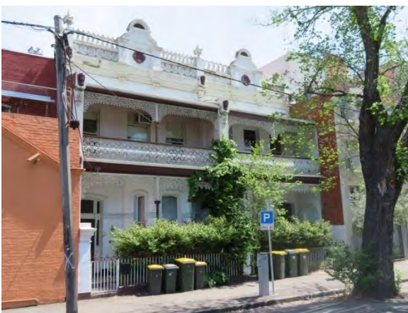
Figure 25 199-201 Cardigan Street, Carlton (HO32) Source: Lovell Chen
