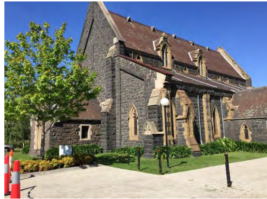
Figure 12 South Yarra Presbyterian Church, 621 Punt Road, South Yarra (HO6) Source: Lovell Chen
