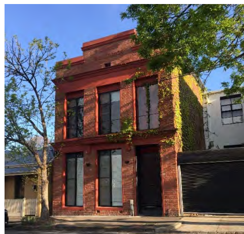
Figure 13 49 Owen Street, Carlton (HO1) Source: Lovell Chen
