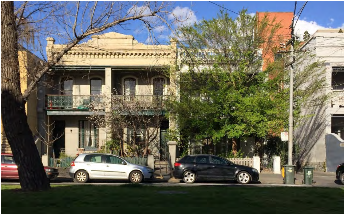
Figure 10 112-114 Drummond Street on the left and 110 Drummond Street on the right concealed by the tree
