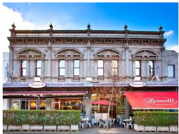
Figure 24 Shops at 198-204 Faraday Street, Carlton, (HO1) Source: Pinstrest
