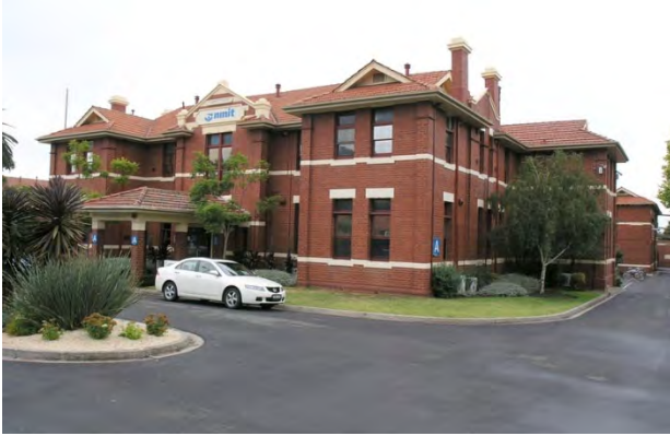
Figure 12 Fairfield Hospital (former) (H1878) Source: Victorian Heritage Database
