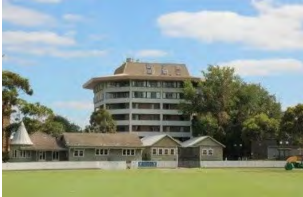
Figure 12 McCaughey Court at Ormond College, HO323 Source: Pintrest
