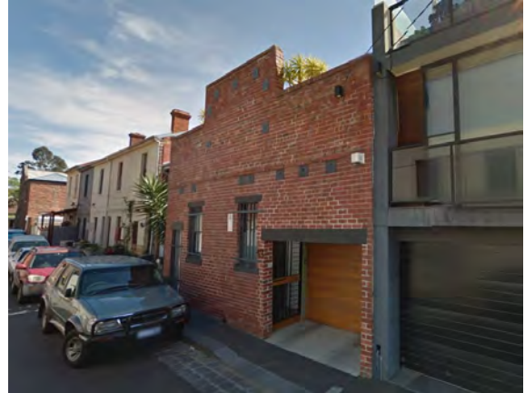
Figure 9 13-23 David Street, Carlton (HO1) Source: Streetview
