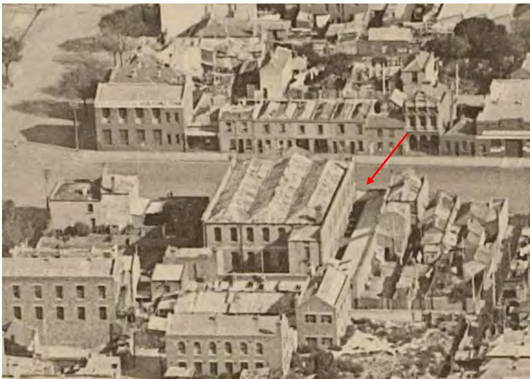
Figure 7 Detail of oblique Airspy view of Carlton, 1927, showing rear (north) of warehouse; the vehicle (carriage gate) entry and driveway on the west side (indicated) has been roofed over by this time, as per the current condition Source: Airspy collection, H2501, State Library of Victoria
