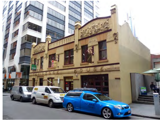
Figure 12 Tavistock House, Flinders Lane Melbourne (H0787 and HO648) Source: Victorian Heritage Database
