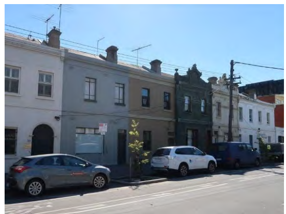
Figure 12 101-111 Cardigan Street, Carlton (HO30) Source: Lovell Chen
