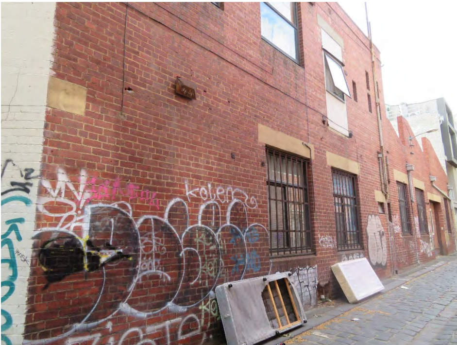
Figure 17 144-146 Queensberry Street, Carlton viewed from Queensberry Lane
