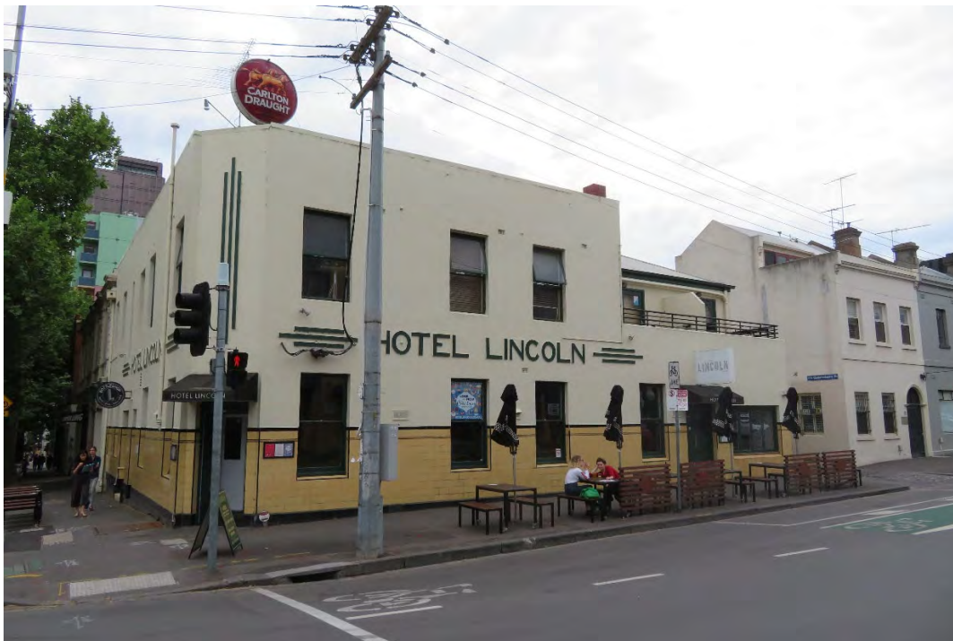
Figure 13 Hotel Lincoln viewed from the intersection of Queensberry and Cardigan streets Source: Lovell Chen
