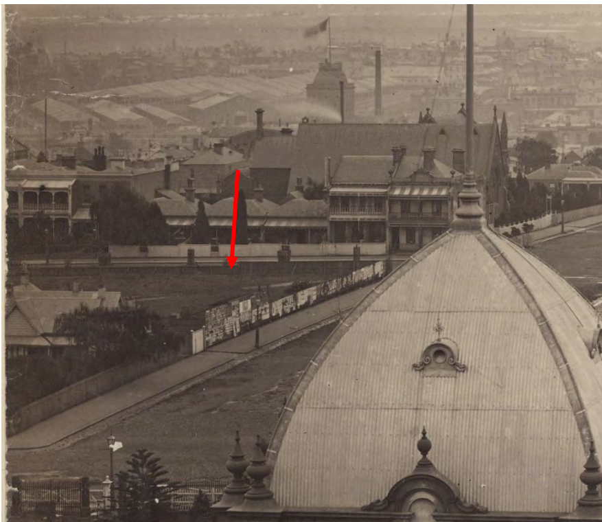
Figure 3 View of intersection of Rathdowne and Queensberry streets, c. 1880s, with subject site indicated (prior to construction of the dwelling) Source: Photographer unknown, H4570, State Library of Victoria
