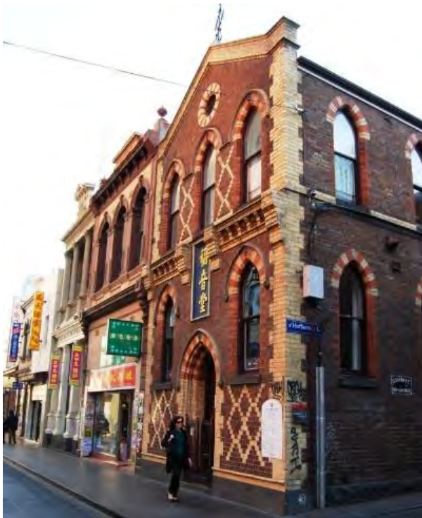
Figure 28 Chinese Mission Church, 196 Little Bourke Street, Melbourne (1872, HO507)
