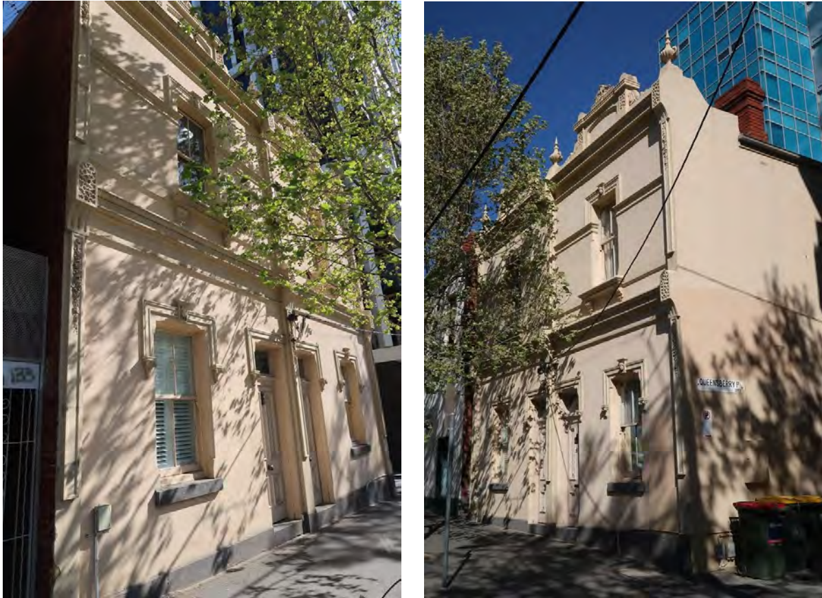
Figure 7 133-5 Queensberry Street from the north-east (at left) 133-5 Queensberry Street from the north-west (at right) Source: Lovell Chen
