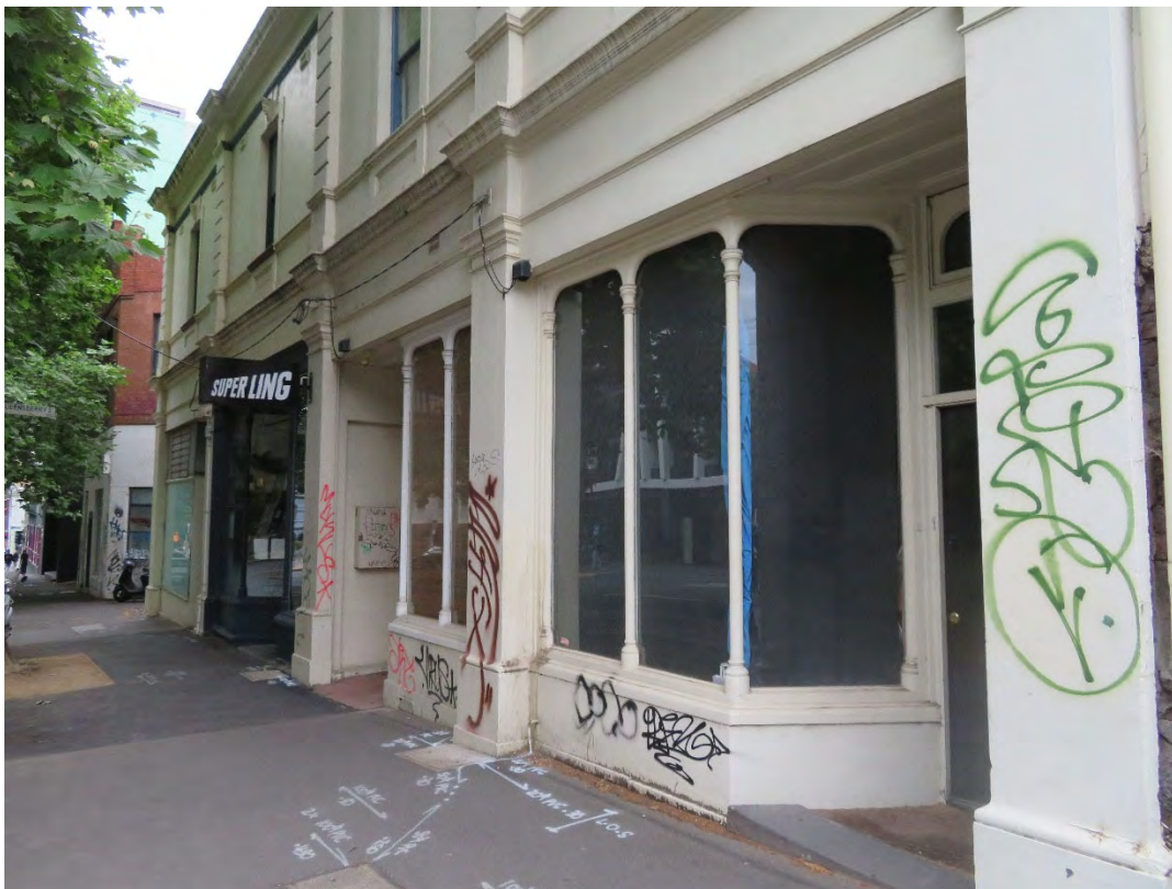
Figure 14 Nos 134-6 (foreground) and 138-40, Queensberry Street Source: Lovell Chen
