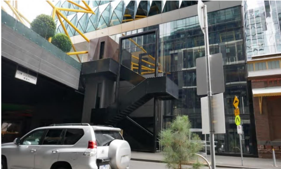
Figure 7: Stair access between Collins Street and Village Street
