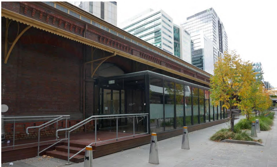
Figure 22: Image of recent alterations and additions to the northern Goods Shed building along Village Street
