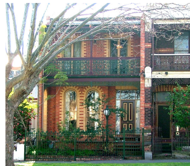
10 Canning Street, North Melbourne
