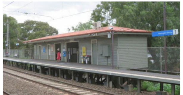
Flemington Bridge Station building and platform south side (up side)
