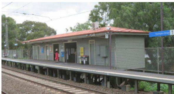
Flemington Bridge Station building and platform south side (up side)
