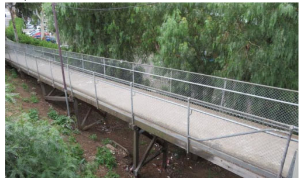
Flemington Bridge Station ramp to the southern platform
