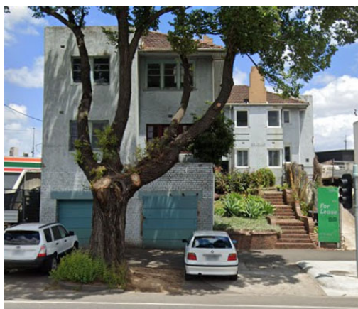
435-437 Flemington Road, North Melbourne
