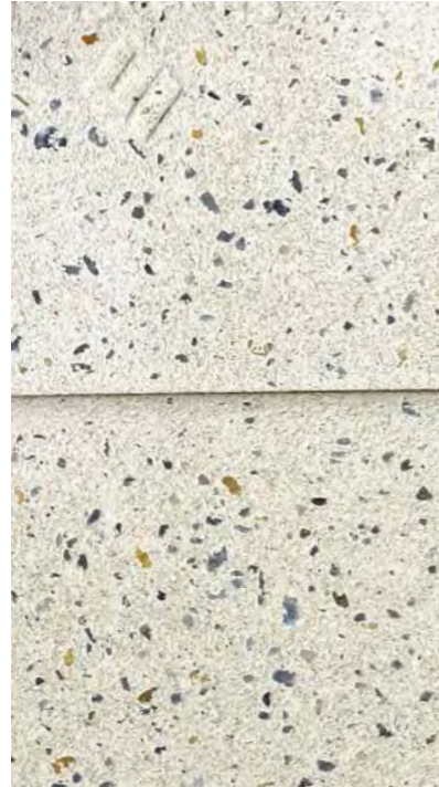
Moulded glass fibre reinforced concrete (GRC) facade grid, with visible aggregate
