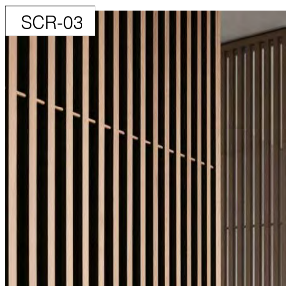
Example of fixed overlooking screening.
