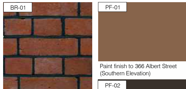
BR-01 Restored brickwork and black pointing finish to 366 Albert Street (Southern Elevation) PF-01 Paint finish to 366 Albert Street (Southern Elevation)
