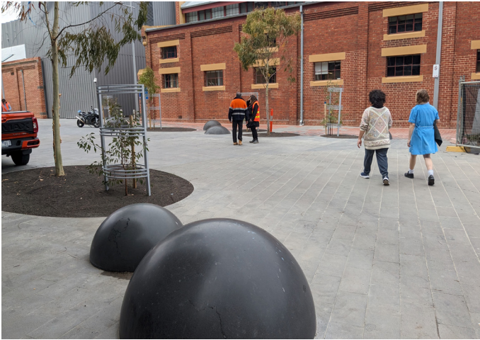
The recently completed bluestone paving
