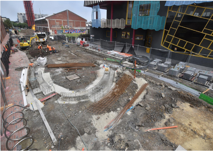
Construction on Dodds Street Linear Park earlier this year
