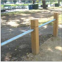
The post and rail fence is used to prevent vehicle access from park perimeters and around car parking areas.
