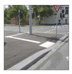
This access ramp detail is for asphalt footpaths at typical street corners throughout the municipality. This detail requires wide footpaths and / or low kerbs in order to maintain preferred slopes and clearances.
