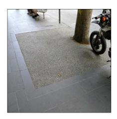
Permeable paving is used for surfacing selected tree pits within the Central City and Docklands. Permeable paving is used with tree pits to allow for the ingress of water and to improve oxygen flow, while providing a stable and easily maintainable surface treatment.
