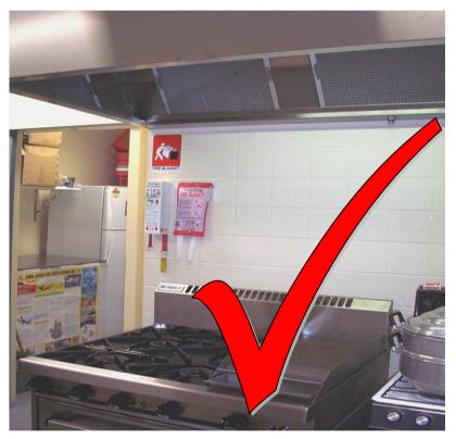
A mechanical ventilation system is required if the energy output is more than 8kW for an electrical appliance or 29Mj/h total gas input for a gas appliance.
