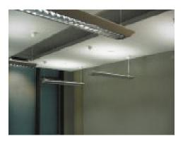
Figure 19. Example of chilled ceiling panel. Source BSEE
