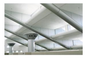
Figure 33. Ventilation stacks, Solar Energy Research Facility, Colorado. Source NREL.
