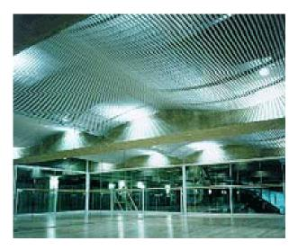
Figure 32. Chilled ceiling panels in Cannons, Covent Garden. Source SAS International
