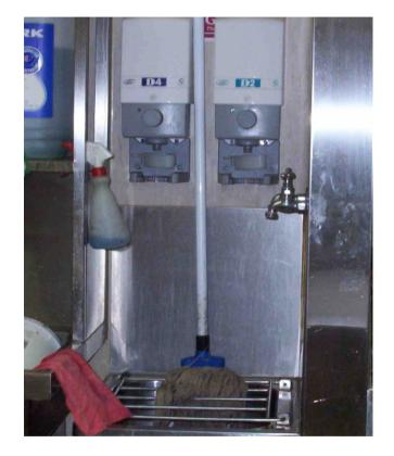
Provide a bin wash or cleaners sink with hot and cold water and connect it to a sewer.
