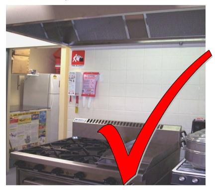
A mechanical ventilation system is required if the energy output is more than 8kW for an electrical appliance or 29Mj/h total gas input for a gas appliance.
