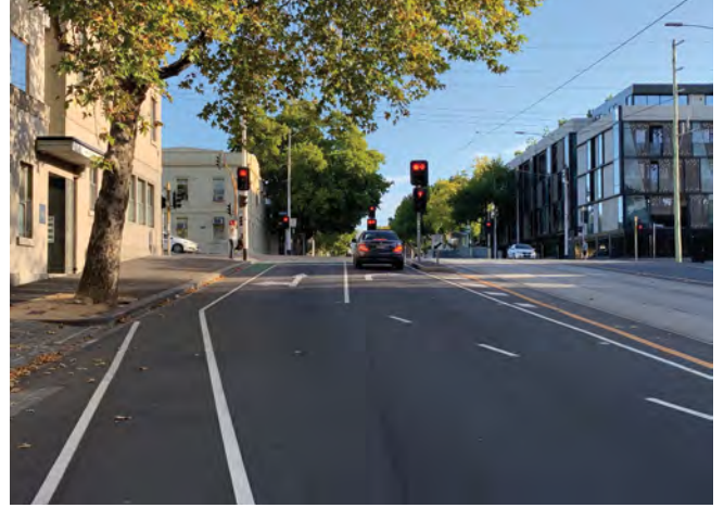
Figure 9: Example of non-physically separated kerbside bike lane - transition from mid-block treatment (top image) to intersection treatment (bottom Image)(Queensberry St, North Melbourne)
