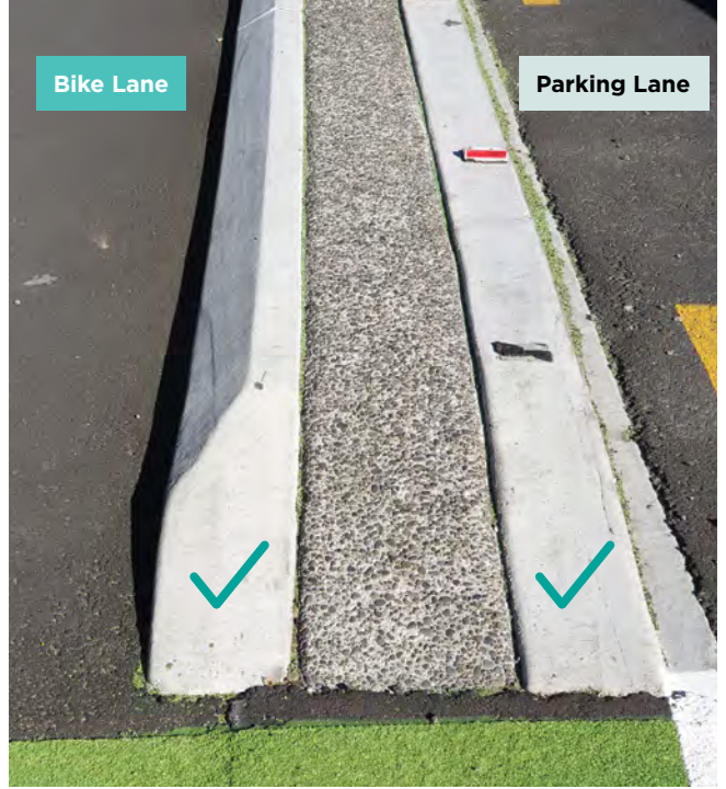
Semi-mountable/Barrier Kerb
