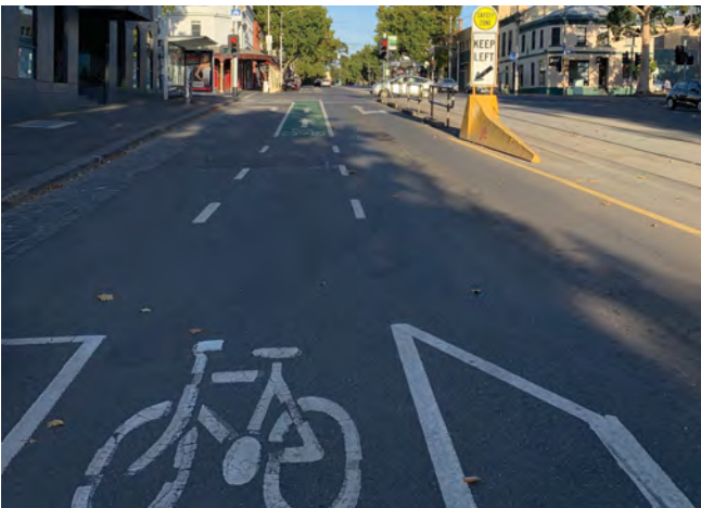
Figure 10: Example of Bike lane between left turn and through traffic lane - transition from mid-block treatment (top image) to intersection treatment (bottom Image)(Queensberry St, North Melbourne)
