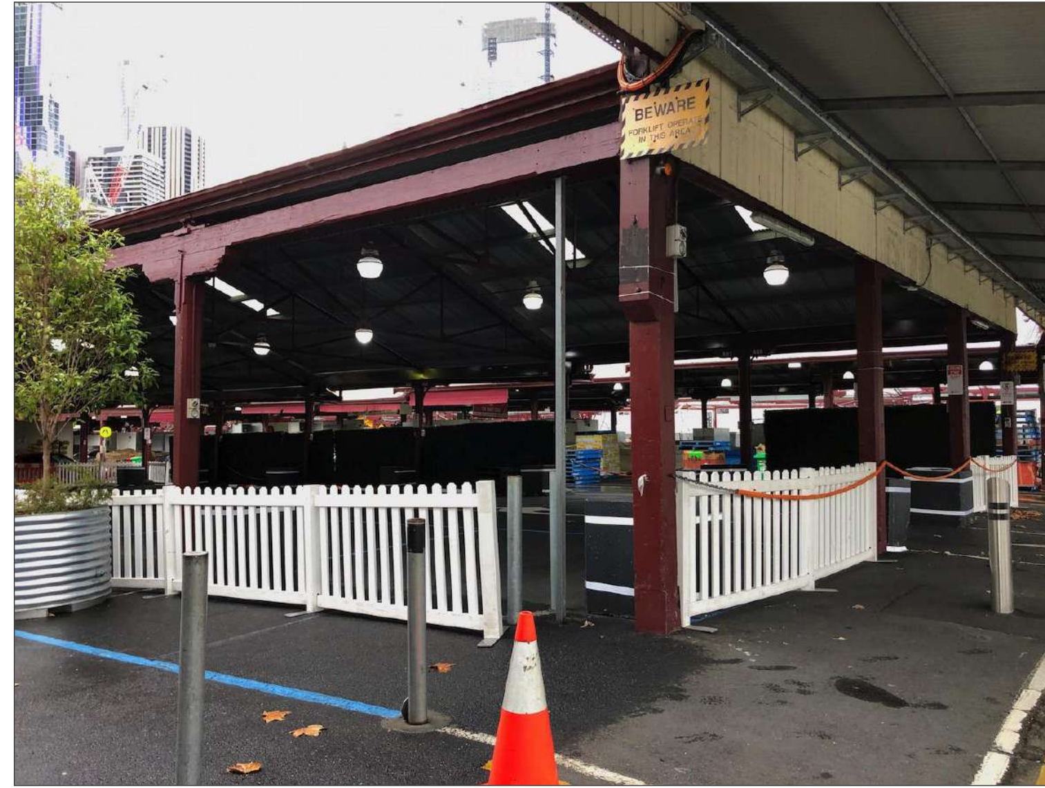
SITE PHOTO 2: SHED A NORTH WEST VIEW
