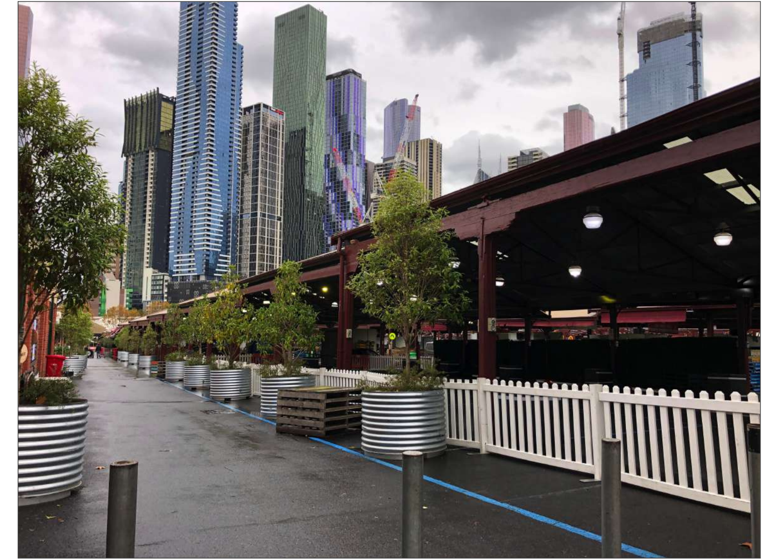
SITE PHOTO 3: SHED A PEDESTRIAN PATH
