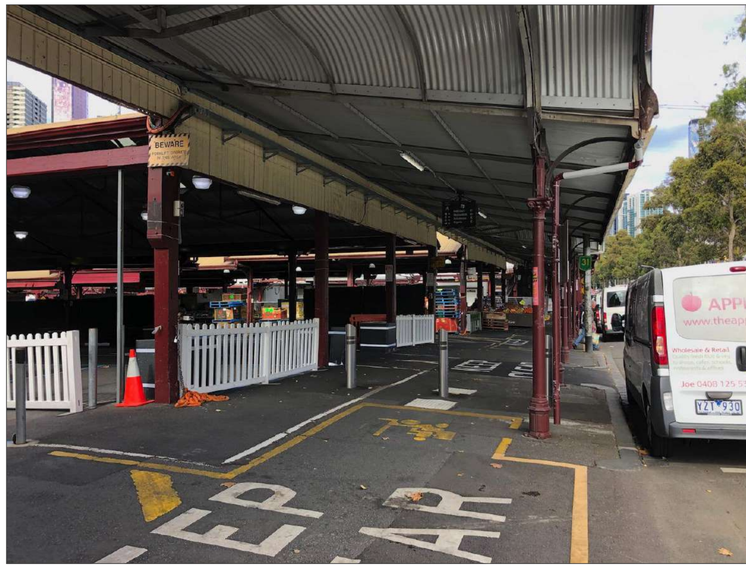
SITE PHOTO 4: PEEL ST PEDESTRIAN PATH NORTH VIEW
