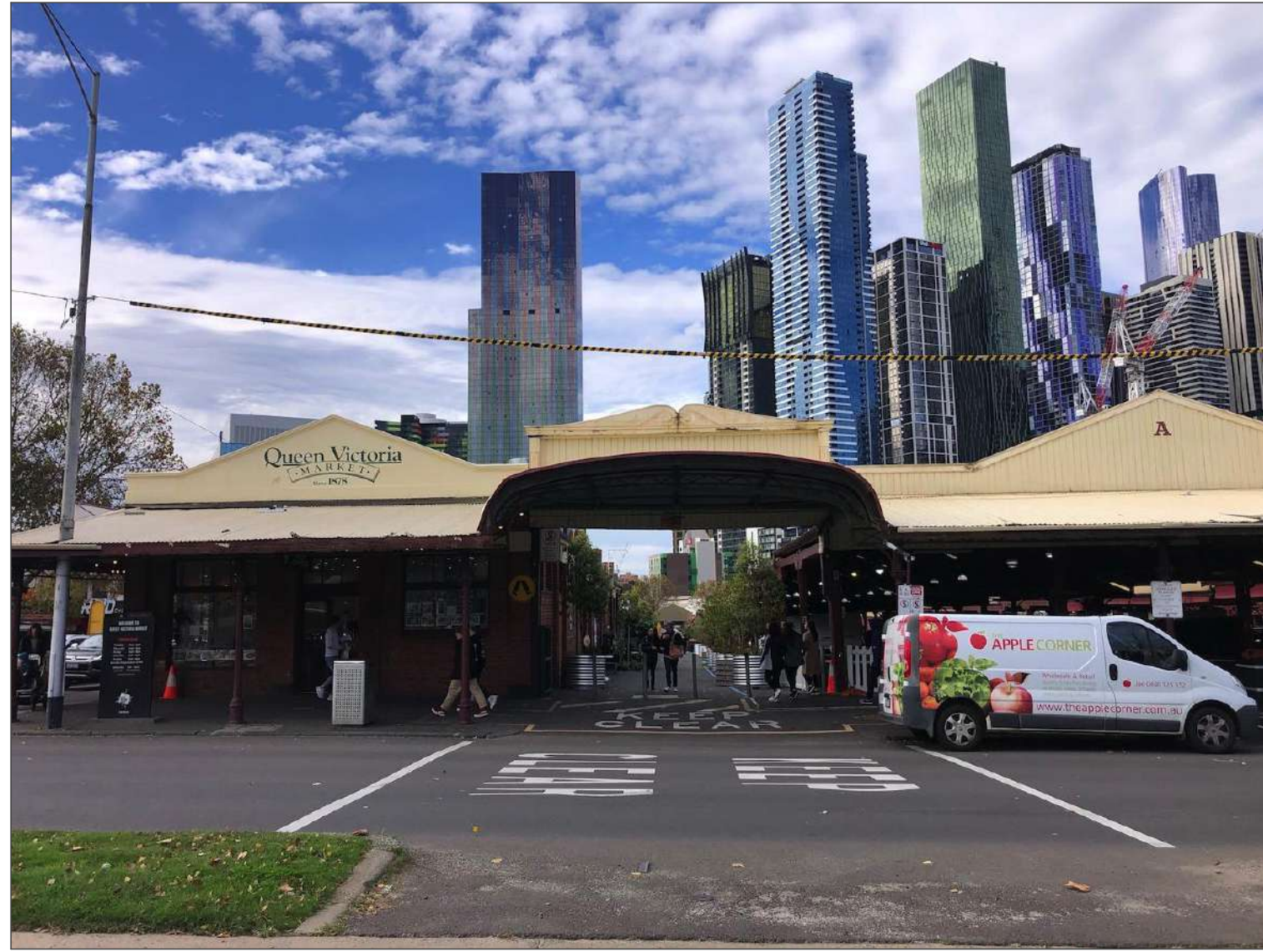
SITE PHOTO 1: SHED A PEDESTRIAN PATH NORTH VIEW
