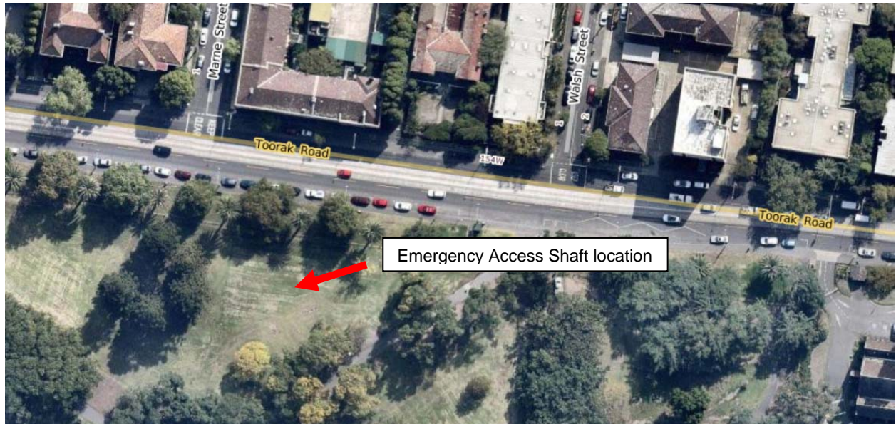
Figure 13 – Emergency Access Shaft location between Marne St and Walsh St alignment (CoMPASS)
