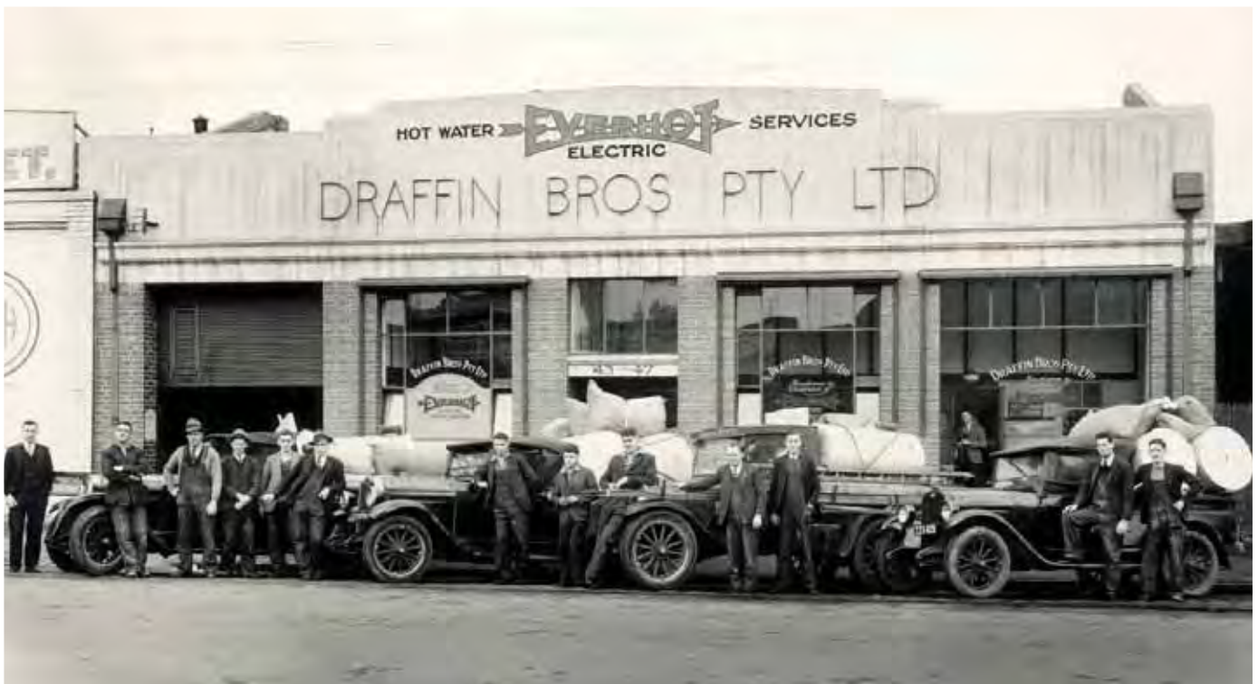
Figure 2.3: Draffin Bros electric hot water service at 43-47 City Road (now Opera Australia) circa 1930s Source: State Library of Victoria
