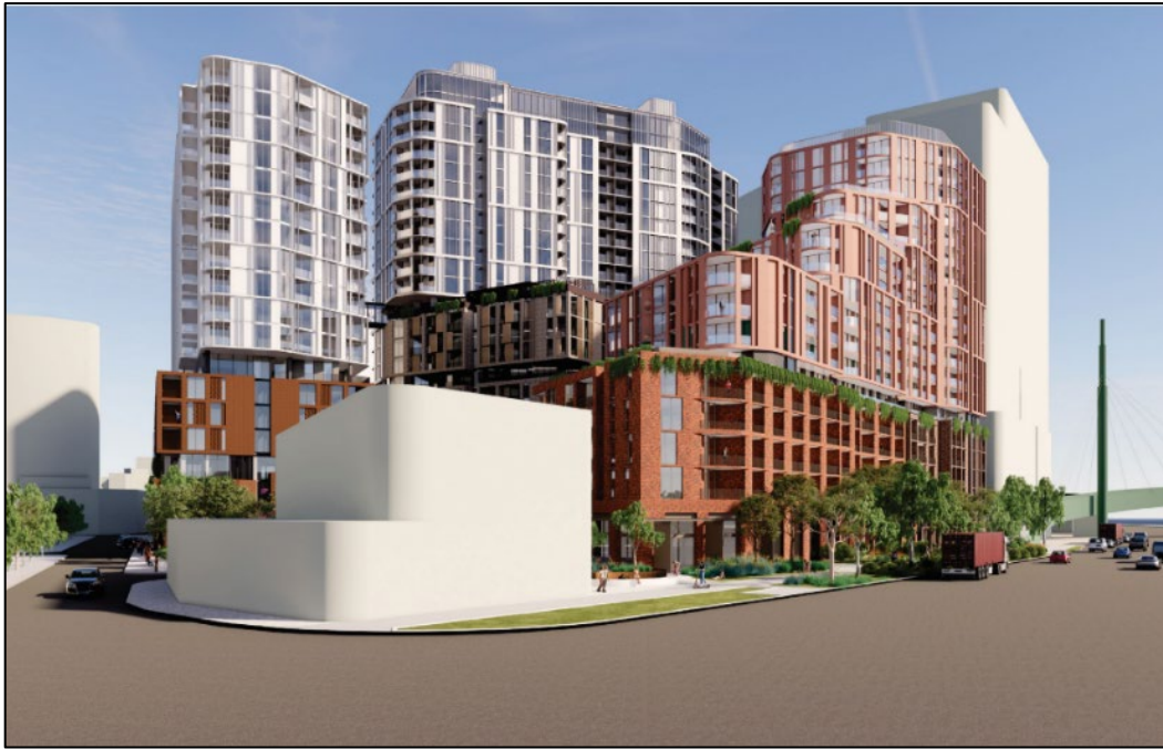
Figure 8 - Buildings 02 and 05 as viewed from the corner of Little Docklands Drive and Footscray Road (source: Urban Context Report)
