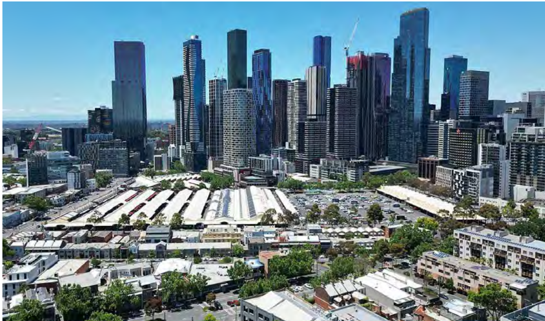
Figure 7: Aerial photograph of the application area from the west looking east
