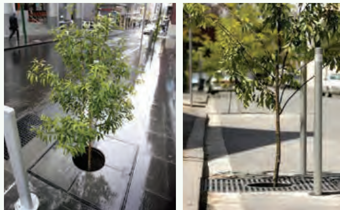
Examples of WSUD tree pits allowing rainwater runoff to increase soil moisture in tree root zones
