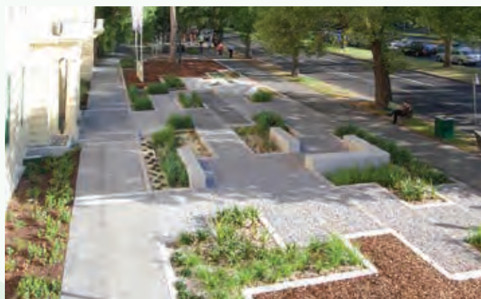
Rain gardens outside the Dame Elisabeth Murdoch Building at the Victorian College of the Arts on St Kilda Rd
