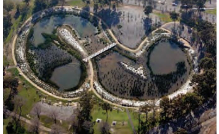
The Trin Warren Tamboore wetland in Royal Park provides habitat, a rich experience for visitors, and captures and cleans stormwater to use for irrigating parkland.
