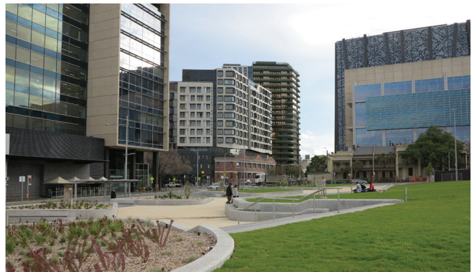
Hard landscape works at the Pelham Street Gateway are now complete.
