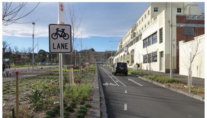
Leicester Street works are now complete and the area is open to pedestrians and vehicles.
