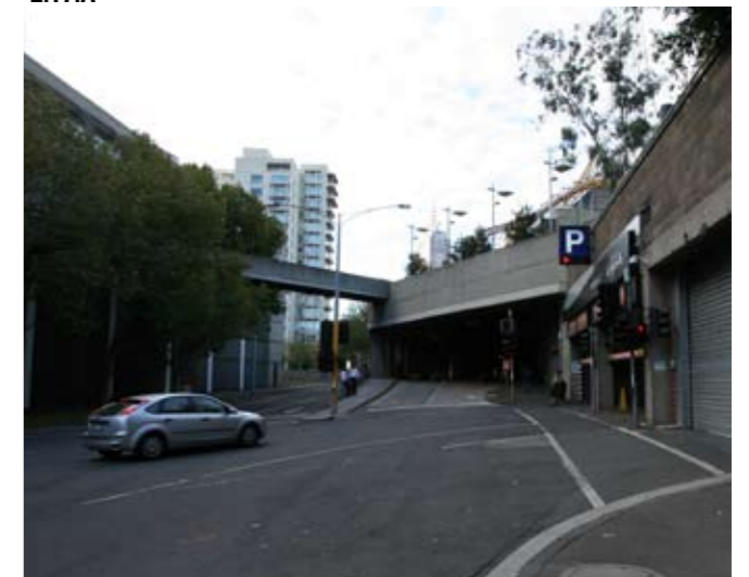
2.17.B Car park entrance at Arts Centre
