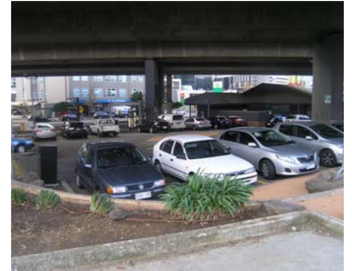
2.17.E Commercial parking under Westgate Freeway
