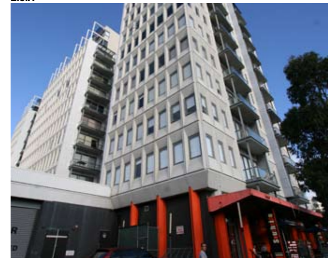
2.6.B Residential Apartments
