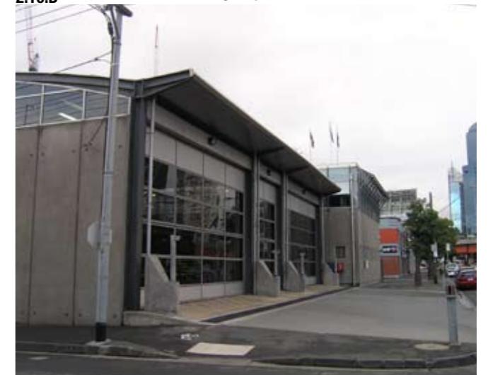
2.10.C South Melbourne Fire Brigade
