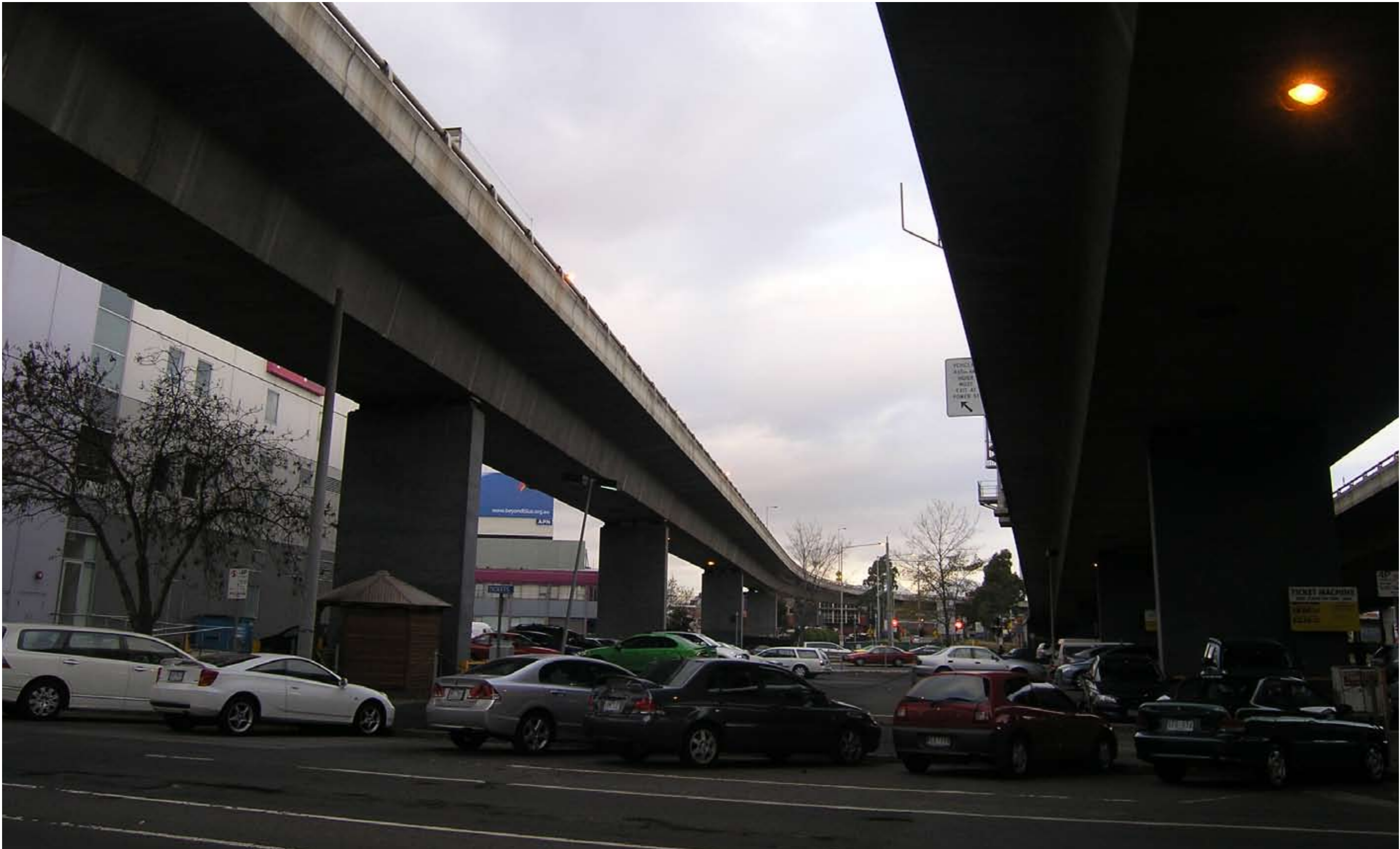
2.17.D Westgate Freeway & Commercial Parking condition
