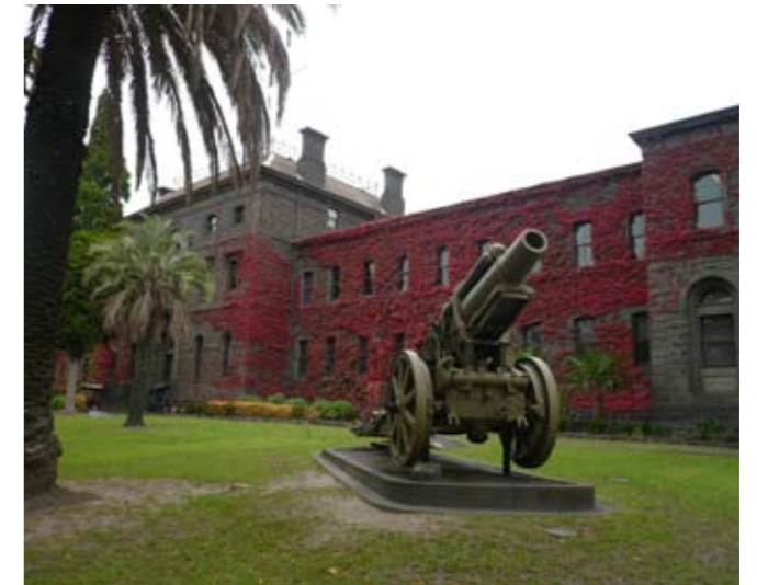
2.4.A Victorian Barracks
