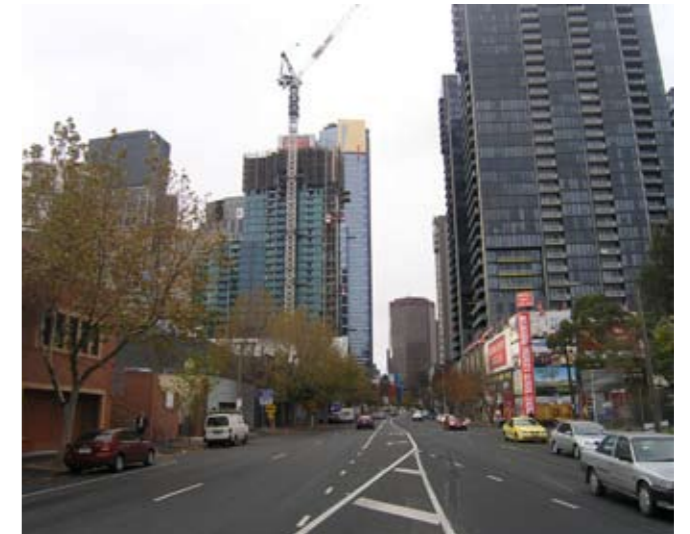
2.13.A View along City Road to Eureka Tower
