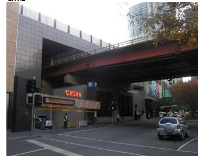
2.17.C Kings Way over Crown Casino car park entrance
