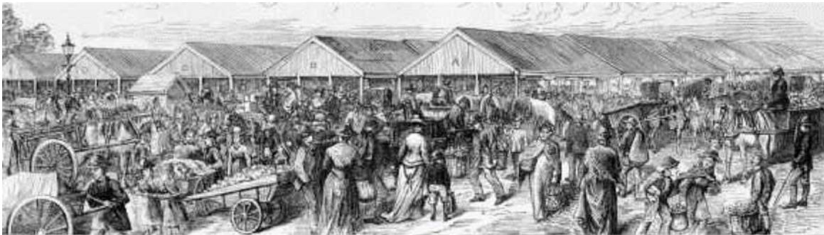
Figure 16 The Queen Victoria Market, showing A to E sheds shortly after construction, 1878
