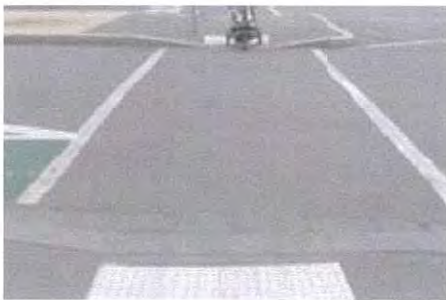
ACCESS RAMP FOR MEDIAN/ISLAND Design Standard 401.04
