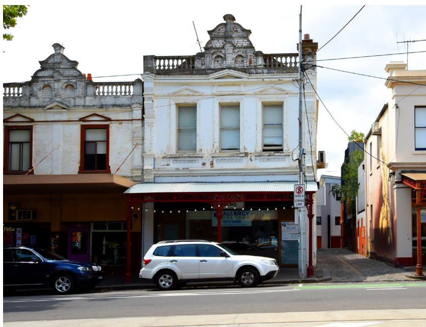
Figure 6 550 Queensbury Street before and after awning reconstruction.
