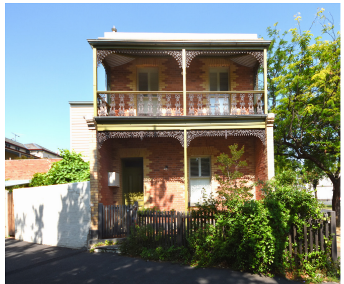
Figure 8 Morrah Street, Parkville - before and after paint removal
