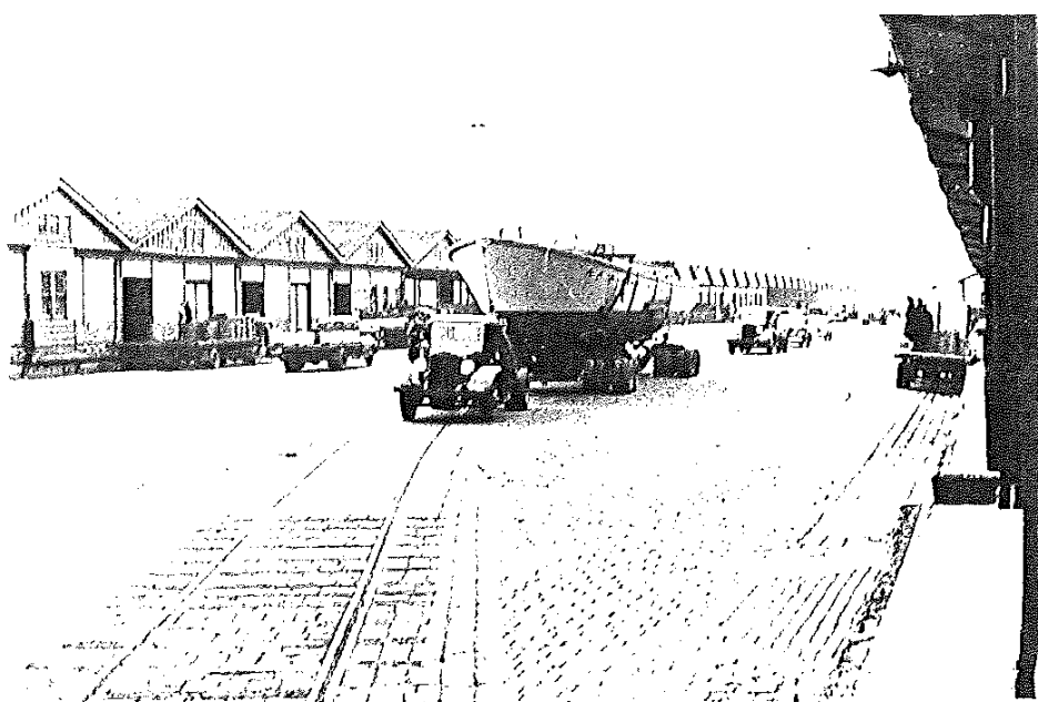
Vessel being transported along North Wharf Road prior to being launched by the steam crane. Notice the "Telford" pitching and rail siding, which remain today.
