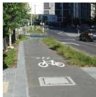
Raised separated bike lane
