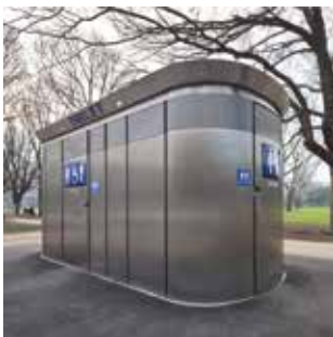
A typical self-cleaning toilet
