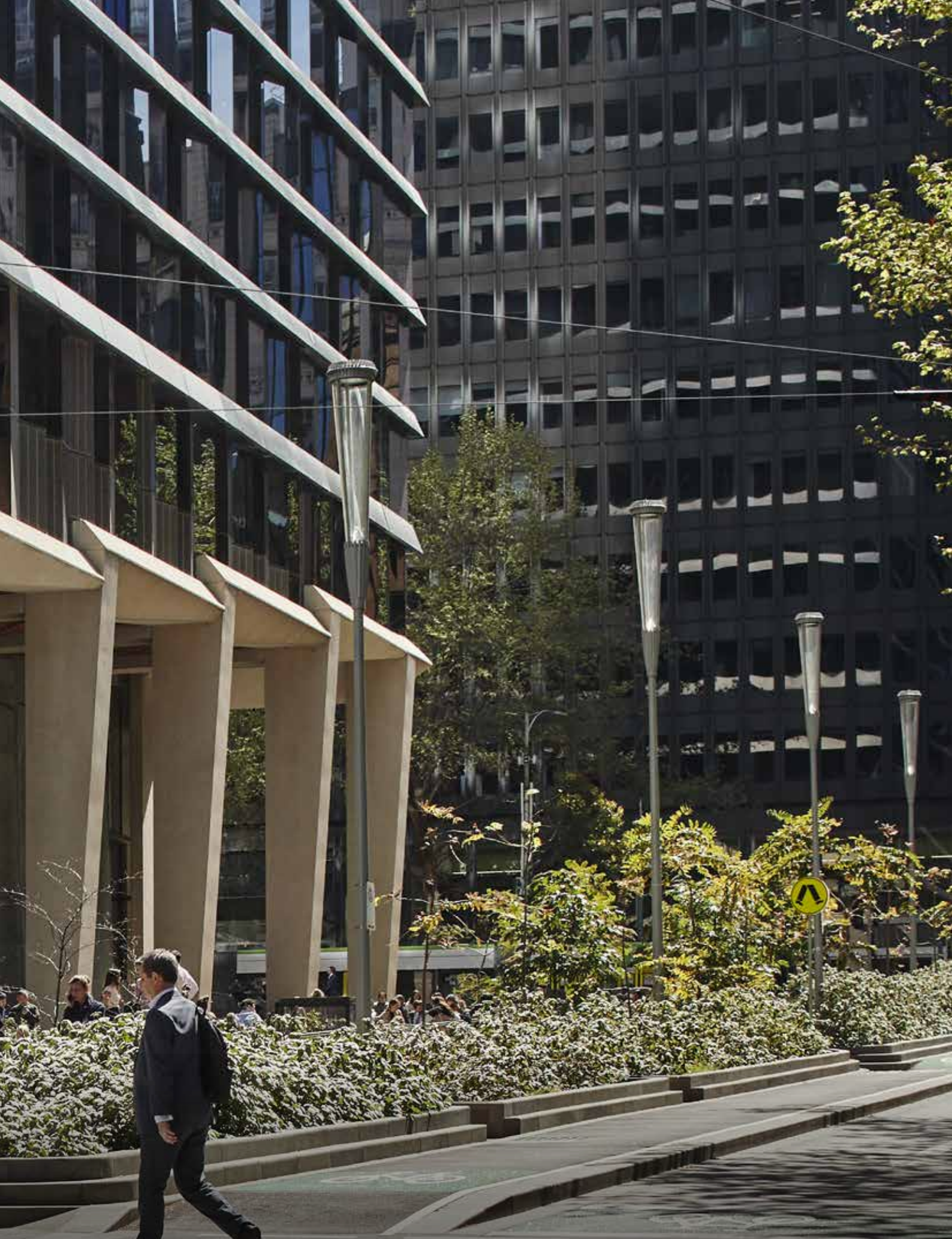
Collins Arch & Market Street Park Photographer credit: Peter Bennetts Design team: Woods Bagot and Oculus Client: Cbus Property and City of Melbourne
