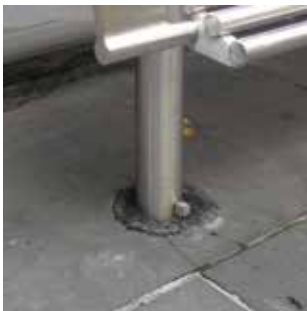
A seat installed into a gib key socket.
