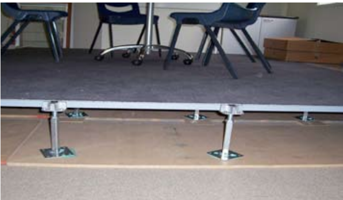
Figure 7. Prototype full scale of the office spaces raised floor
