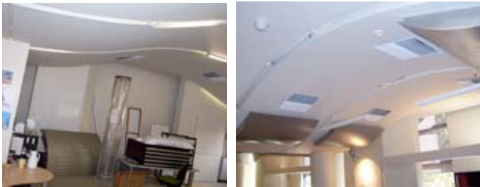
Figure 6. Prototype full scale of the office spaces with precast concrete ceiling-floor system
