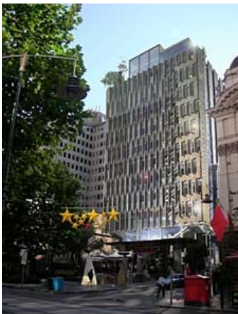
Figure 3. Timber louvred façade to the west which reacts to external conditions and is powered by solar panels (DesignInc Melb)
