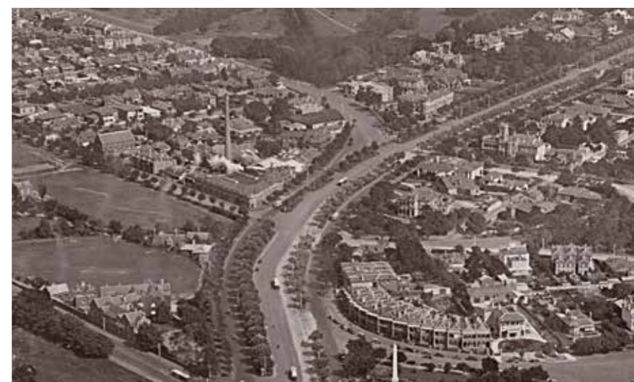
View down St Kilda Road from Domain Interchange to Fawkner Park showing young and mature street trees, taken between 1920 and 1940 [State Library of Victoria].
