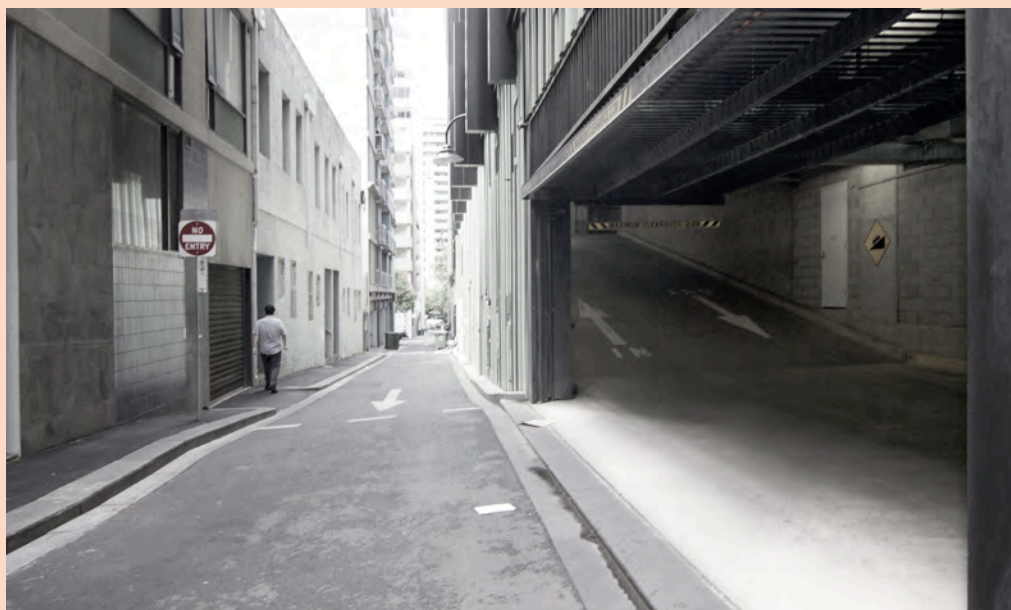
Figure 36 A carpark reliant on ramped floor plates is more difficult to adapt in the future.
