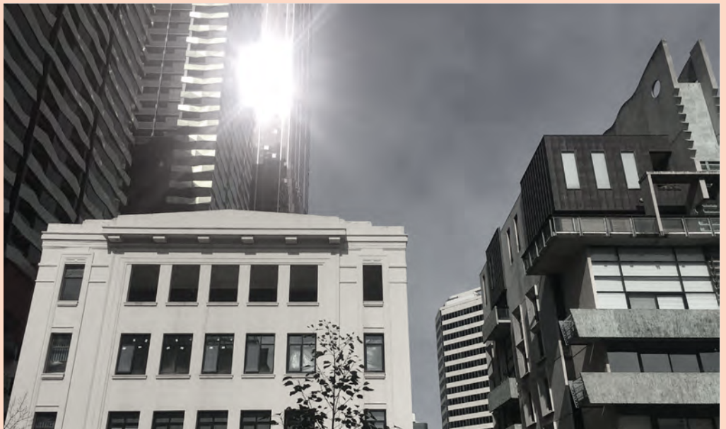
Figure 58 This faceted, highly reflective glass facade without any projecting fins or recesses maximises the intensity of glare to the public realm.
