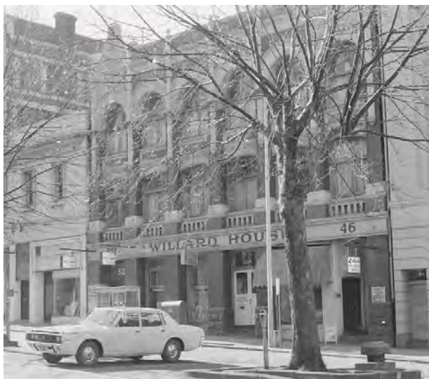
Figure 1. View of the building formerly at 46-52 Russell Street c1972. (Source: Halla 1972, SLV)
