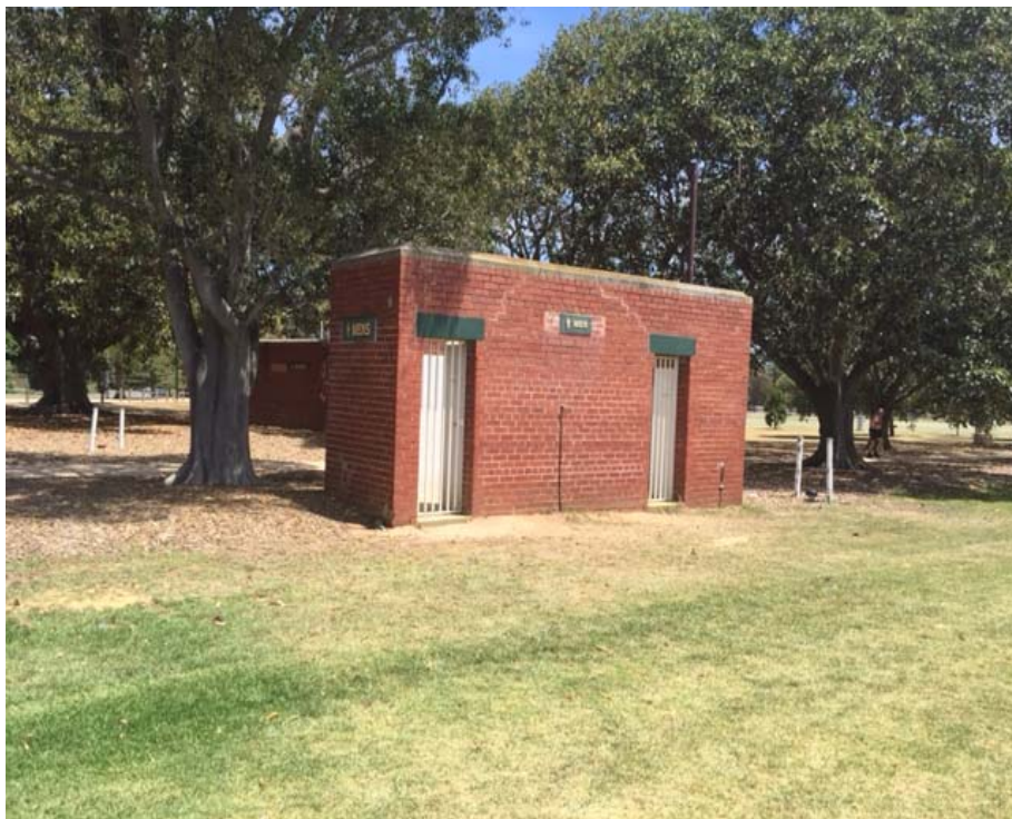
Figure 3: Men toilet blocks. (Photo taken 14 December 2015)
