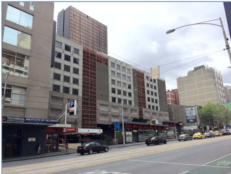
Figure 4: Car park at 224-252 La Trobe Street
