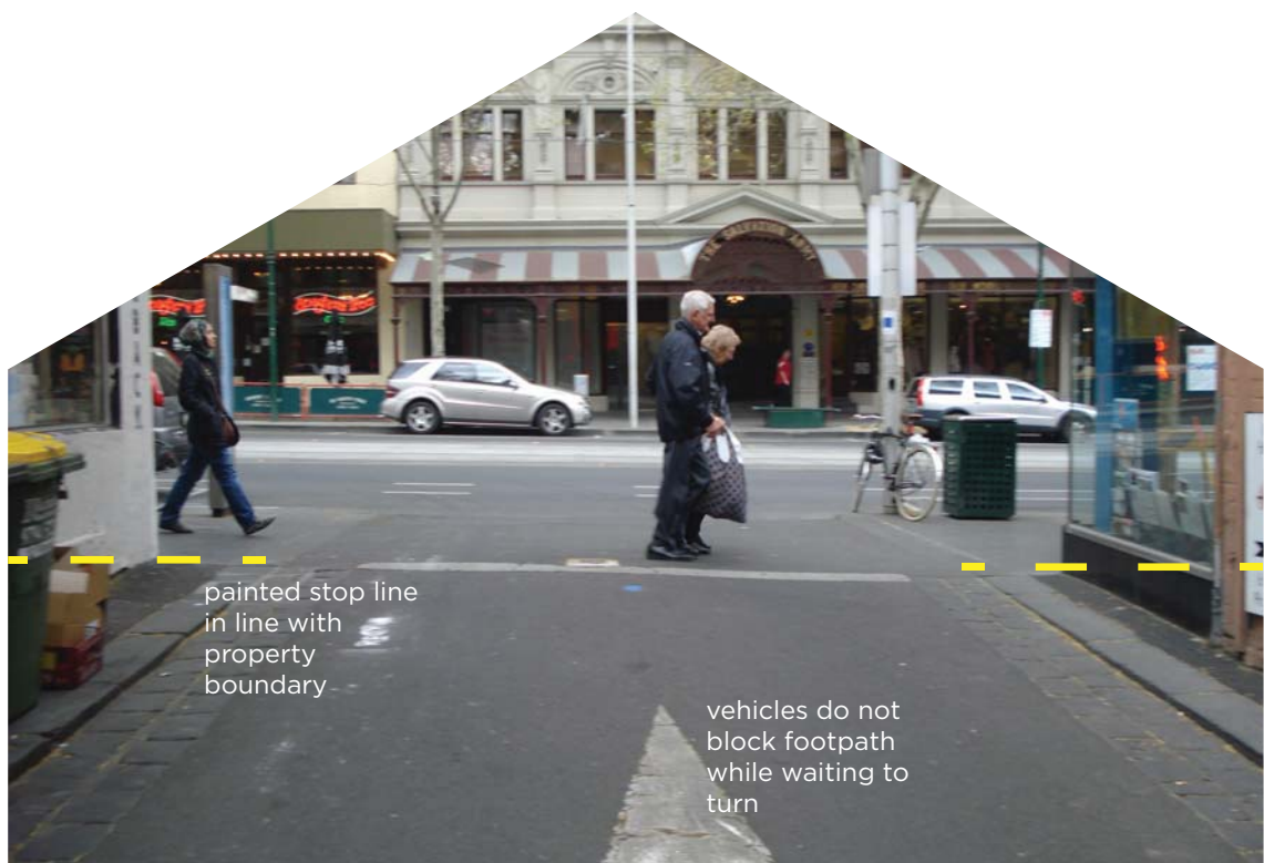
Figure 23: Example of stop line on property line, Crossley Street facing Bourke Street
