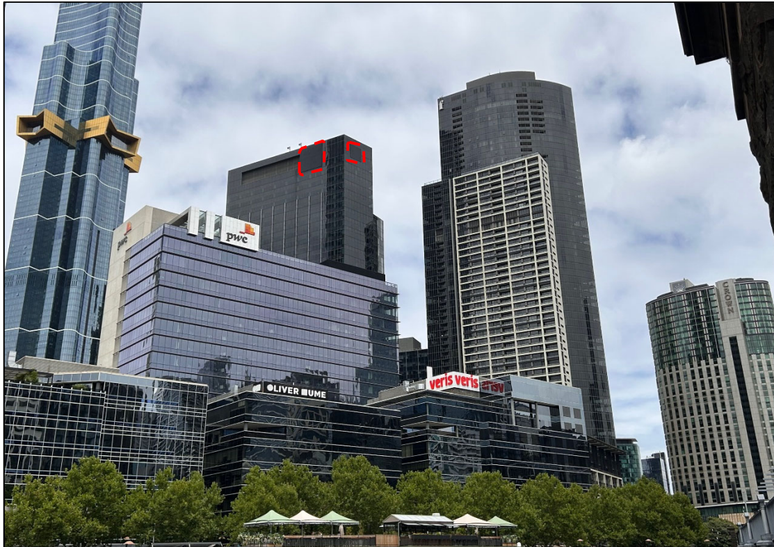
Figure 5. Site showing proposed area of works (in red) – eastern and northern elevation
