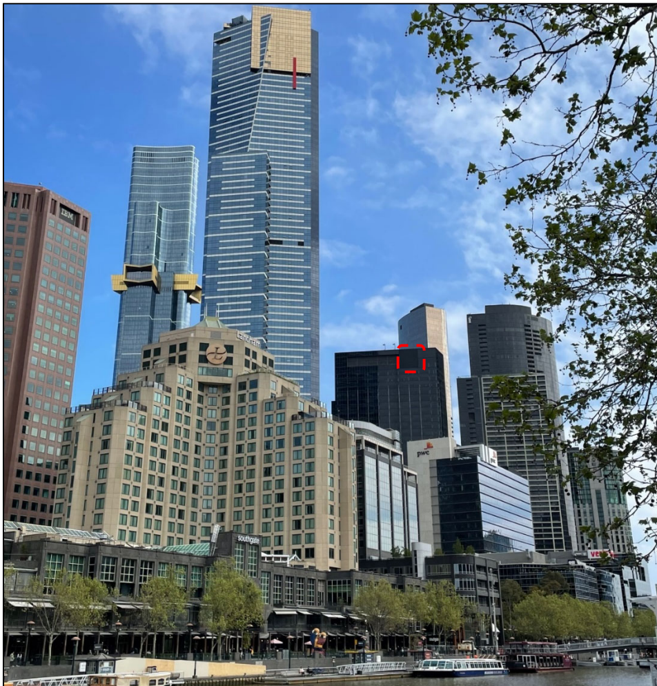
Figure 4. Site showing proposed area of works (in red) – eastern elevation
