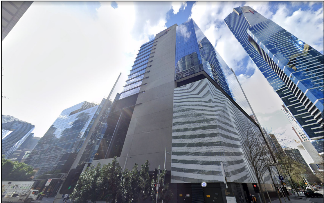
Figure 9. Property located diagonally across to the north-east of the Site at 2 Riverside Quay, Southbank
