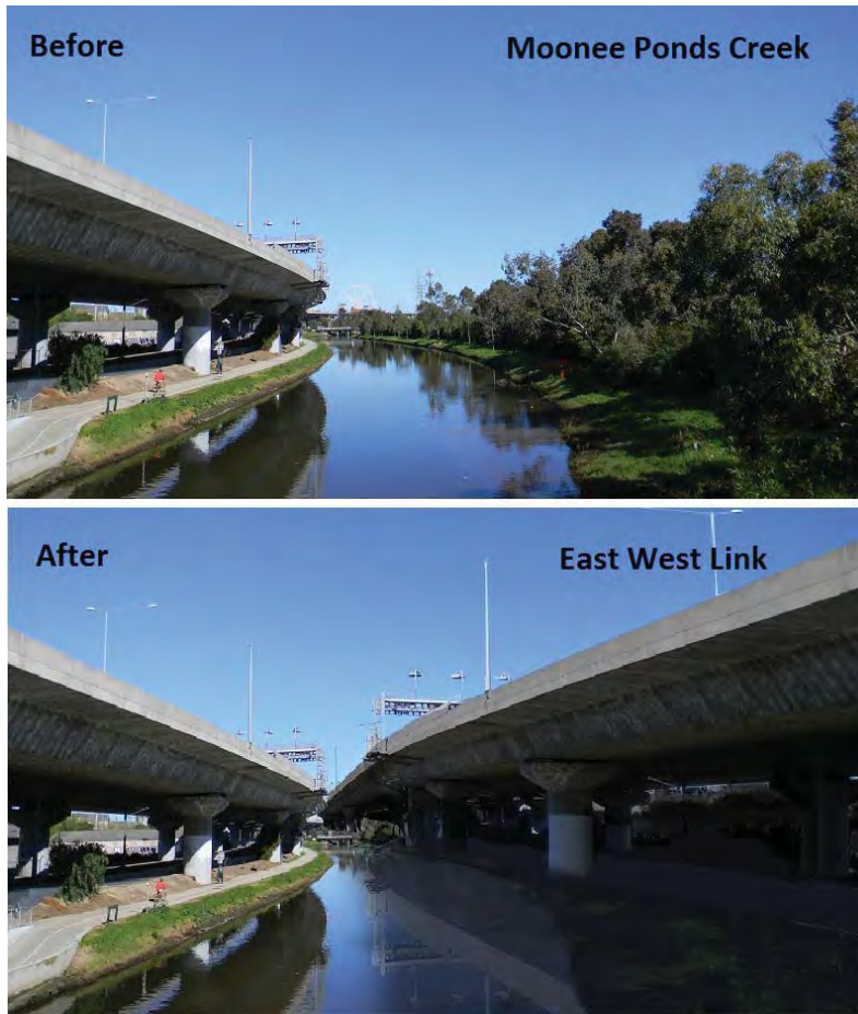
Figure 16: Impact of East West Link on lower Moonee Ponds Creek
