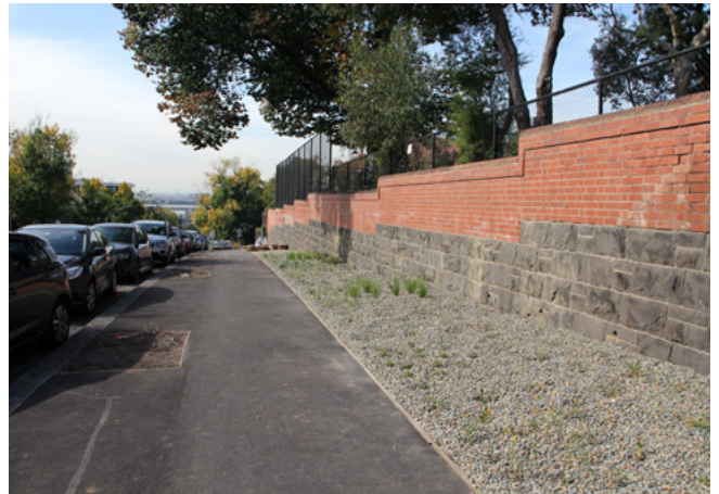
Plant installation (April 2018).
