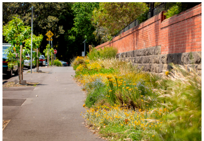
Post-plant installation (November 2019). Photo: David Hannah.
