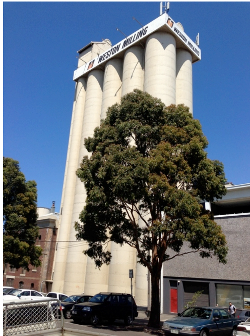
Figure 11 The silos as seen from Munster Terrace.
