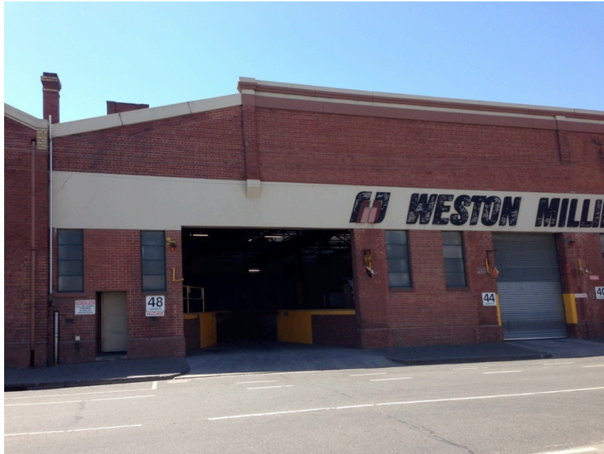
Figure 14 The facade of Building 8, which has been incorporated with the facade to the adjacent Building 1 to the south.
