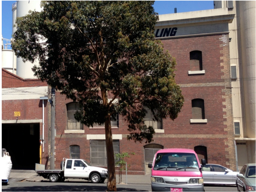
Figure 9 Munster Terrace elevation, with the adjacent silos (Building 5) visible at right.
