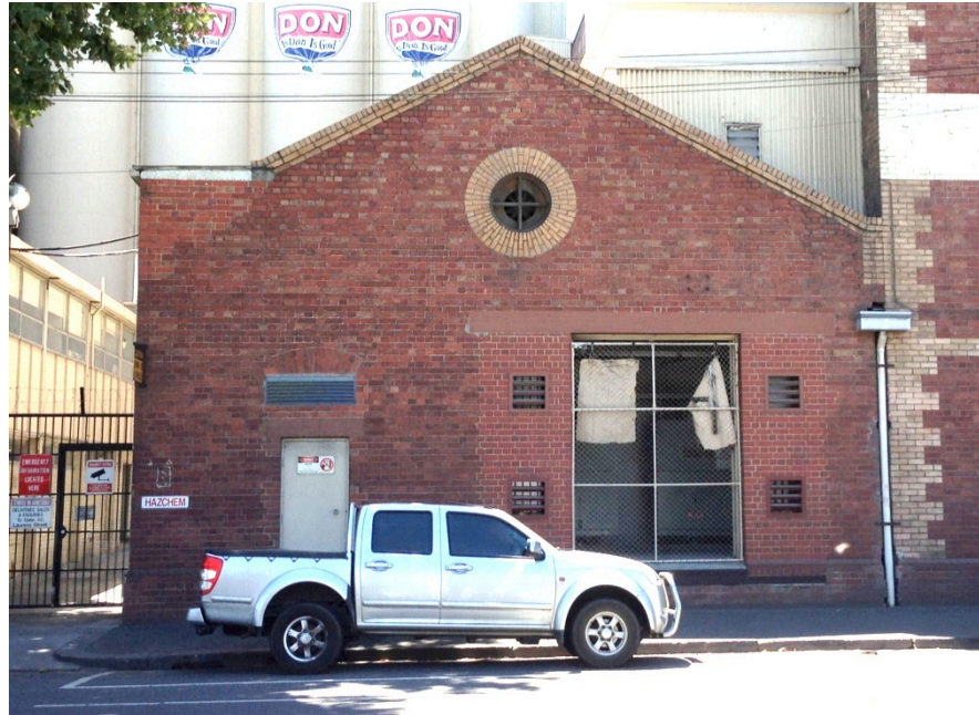
Figure 13 The Laurens Street facade.
