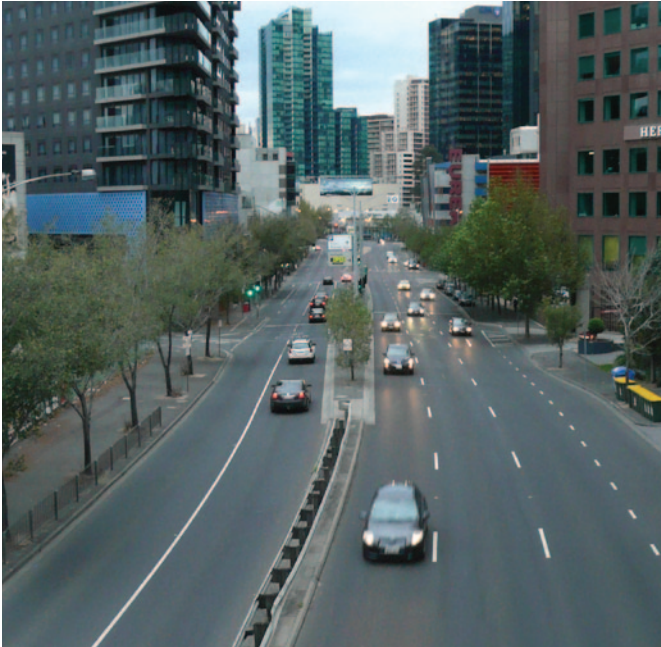
Figure 5.5 Existing condition of City Road
