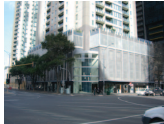
Inactive upper floors of car park podiums
