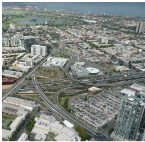
Figure 3.6 Existing CityLink Deck approach
