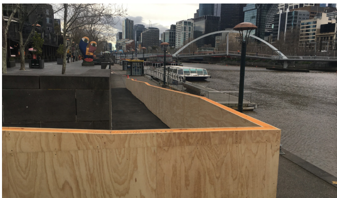
Phase one temporary access ramp
