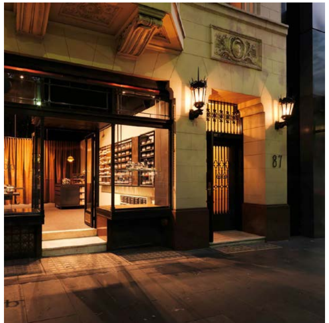
Image 14. Window display lighting and illumination of re-cessed doorways enhances safety. Full details can be found in Appendix 3 - Photo References.
