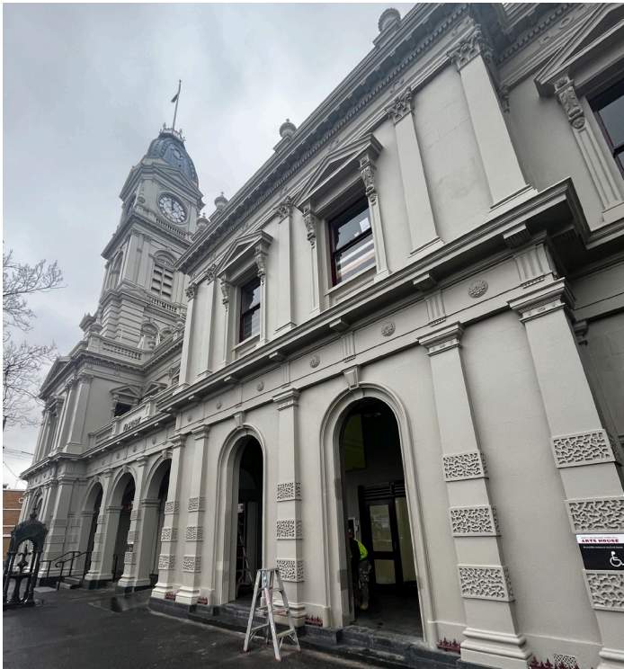
Facade restoration works are now complete
