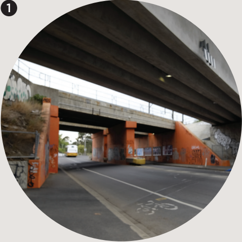
Figure 1.34: Kensington Street railway underpass with poor pedestrian access
