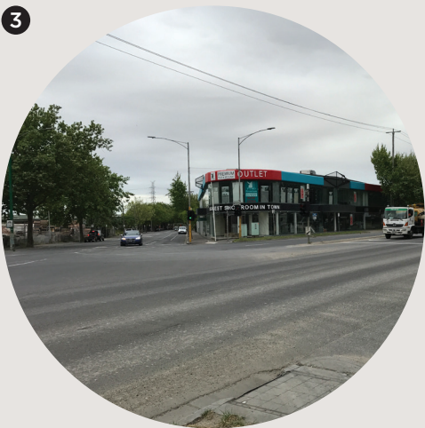
Figure 1.36: Dynon Road and Kensington Road intersection currently being upgraded as part of VicRoads Dynon Road improvements
