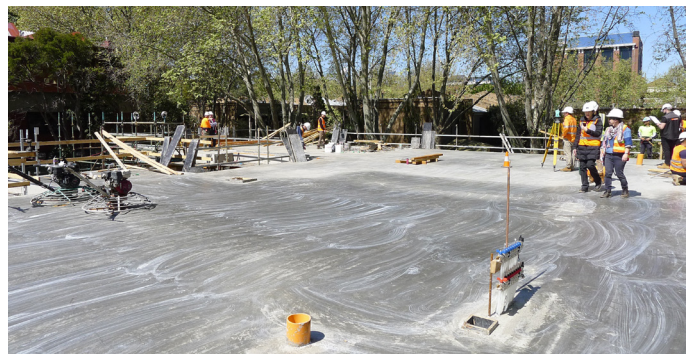
October 2019 - Pour level 1 slab (rear of site)
