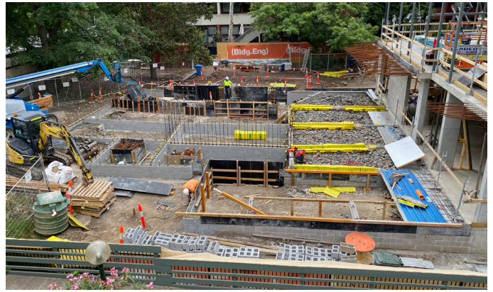
December 2019 – Completion of sub-floor (front of site)
