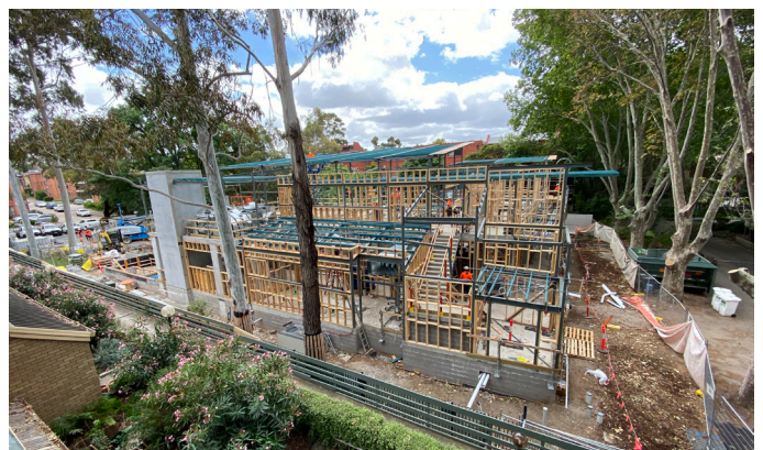
November 2019 - Level 1 roof framing (rear of site)
