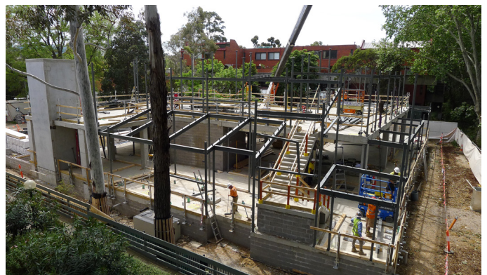
November 2019 - Level 1 column framing (rear of site)
