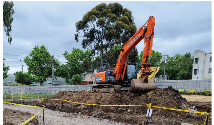
Excavation and soil removal works are underway
