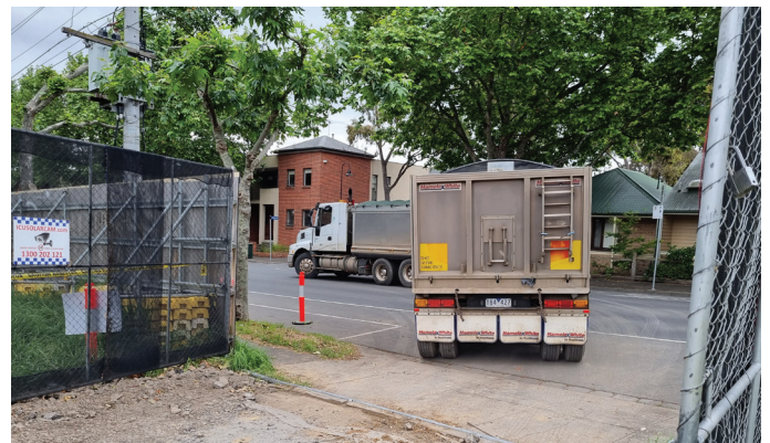
Loaded trucks exit the site via Kensington Road
