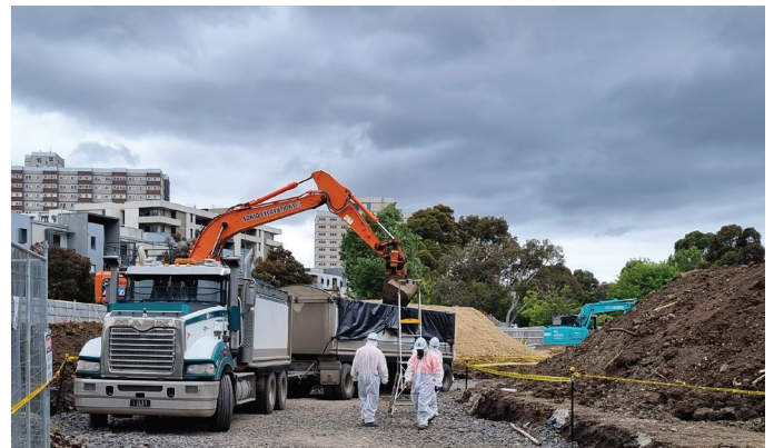
Soil is removed and loaded onto trucks
