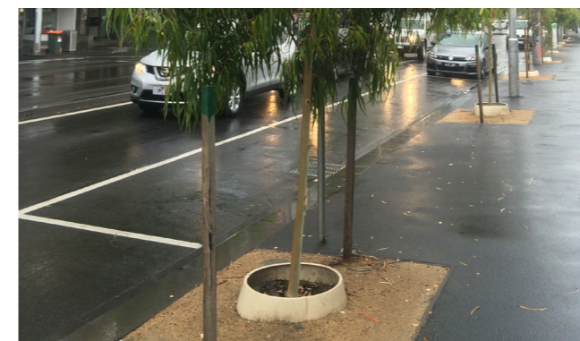
Image 15: Tree replacement soak wells and soil volume (Flinders Street)
