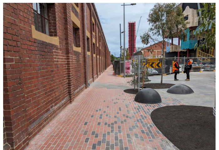
The recently completed paving
