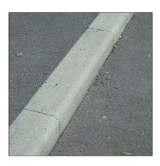
Precast exposed aggregate concrete kerbs are typically used for medians and traffic islands outside the Central City where they are typically installed without a gutterstone.
