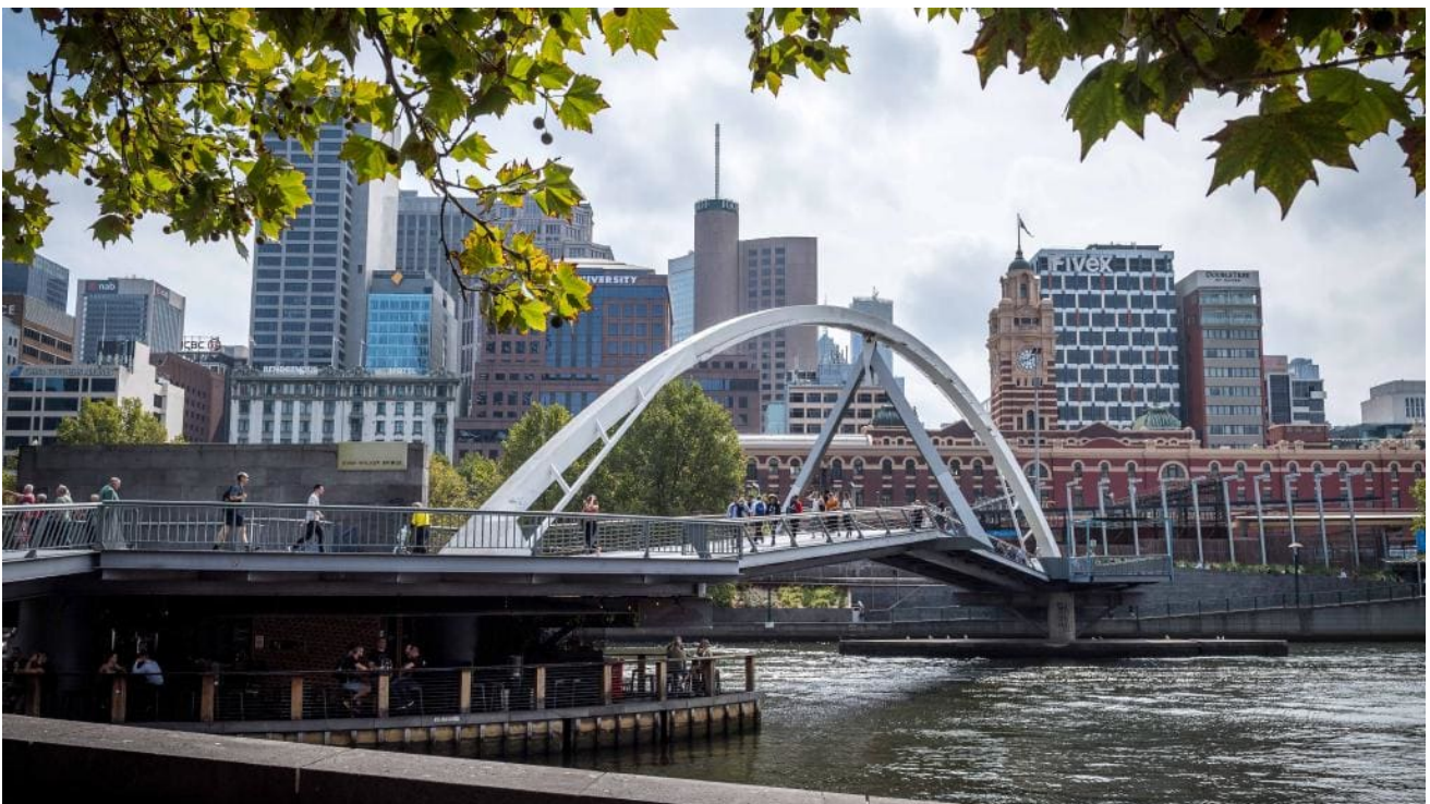
Figure 2: The Yarra Footbridge or ‘Evan Walker Bridge’ demonstrates an example of a structure completed in 1992 which was considered to have stood the test of time as an enduring design contribution to the City.
