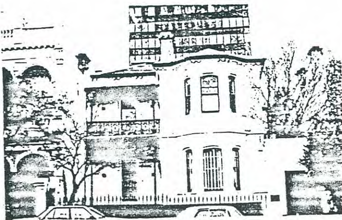
A large freestanding residence in Drummond Street. The hipped slate roof, seen in the earlier period, is still used although the decorative wall elements are more numerous and complex. The cast iron balcony was almost universal in Carlton in this period although this configuration with a projecting bay window was more common in other areas.
