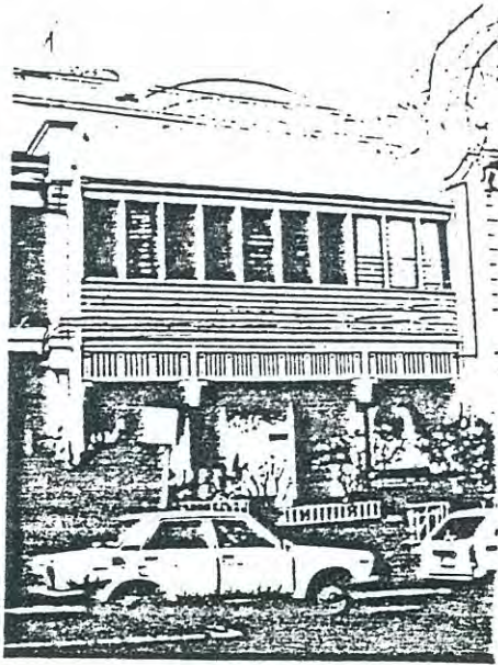
Development in Carlton in the Edwardian period was limited and this example shows a typical Victorian form still in use albeit with later art nouveau decoration. Other Edwardian features include the timber frieze and assymetrical disposition of ground floor fenestration.
