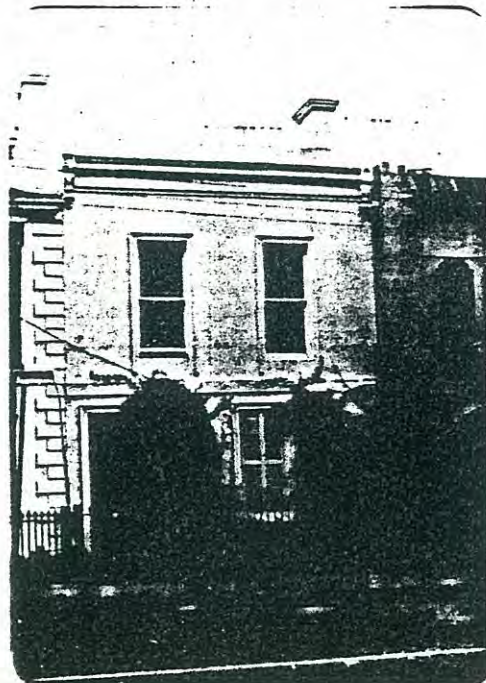
A restrained parapet, simple architrave moulding around windows and doors, and timber shutters were common early Victorian architectural details. The austere facade without verandah was also typical although this example once has a verandah cantilevered on decorative timber joists.
