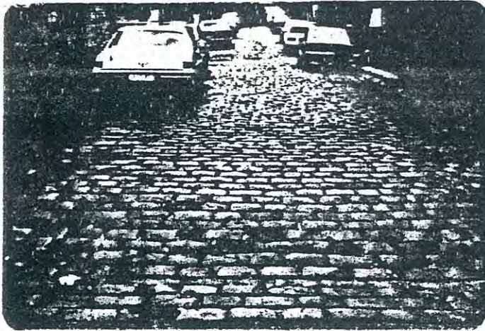
Although Carlton retains a superb network of bluestone laneways, only a handful of bluestone paved streets remain. This example (left) in South Carlton should be retained to demonstrate this once common street surface. Other bluestone
