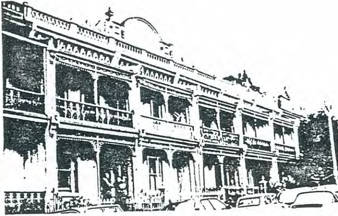
Two large rows of attached terrace houses. Melbourne terrace in Drummond Street has flamboyant decoration on the parapet with use of cast iron balconies while the larger three storey example further up Drummond Street dispenses with cast iron and uses masonry arching as the predominant decorative treatment.
